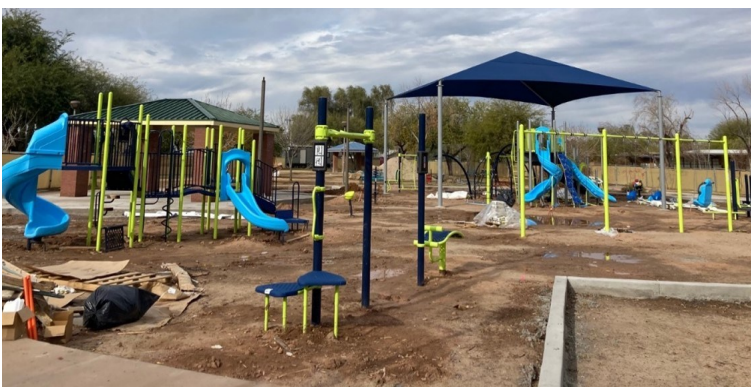
Left: Mitchell Playground Construction
