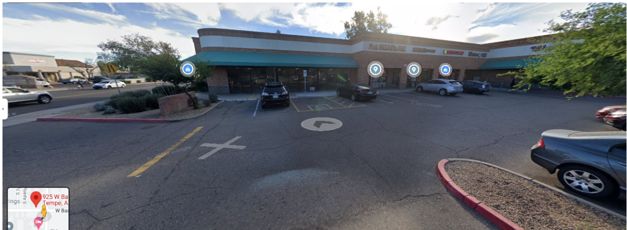
Location: Parking Lot facing south towards storefront
