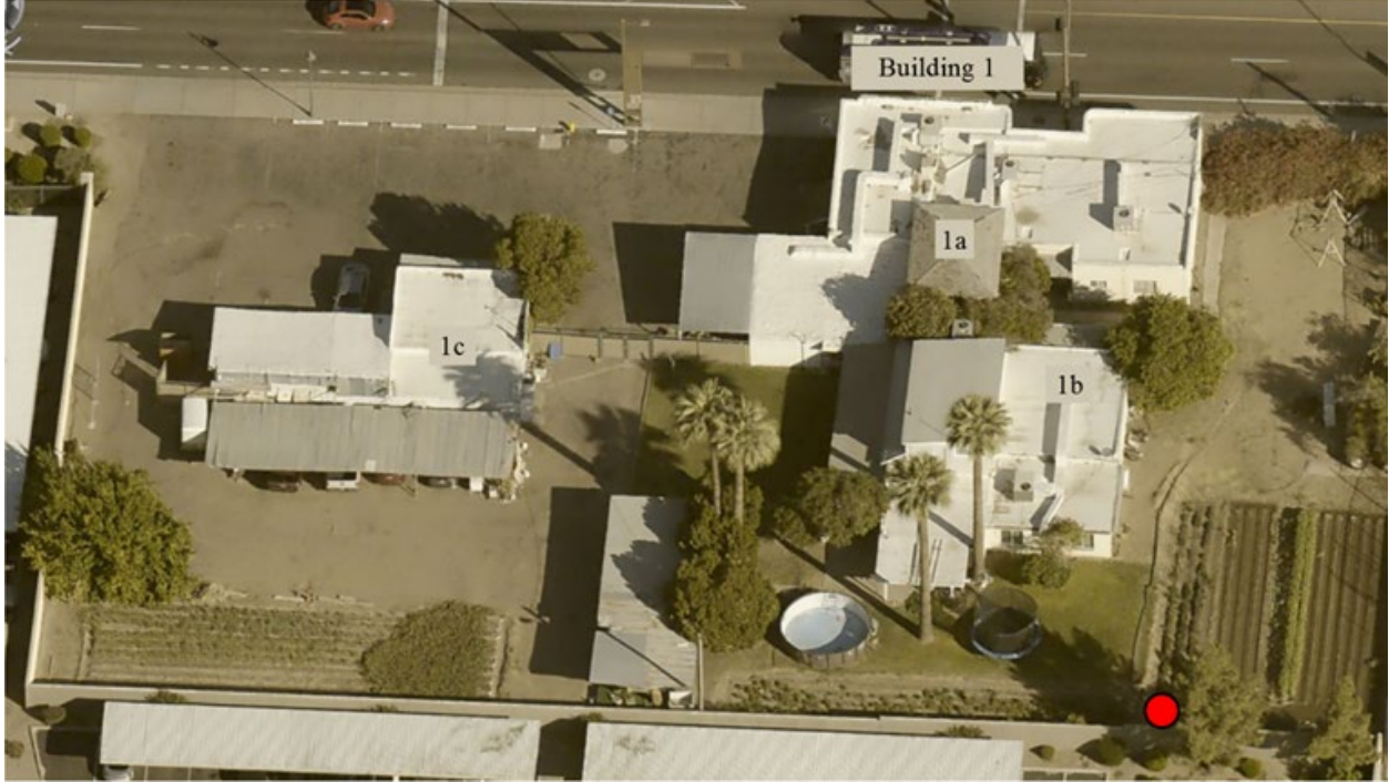
Aerial photograph showing components of Watson's Flower Shop Building 1.
