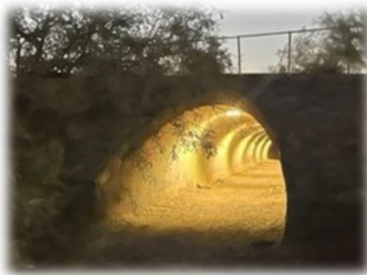
Above Left: Curry Tunnel Lighting Install
