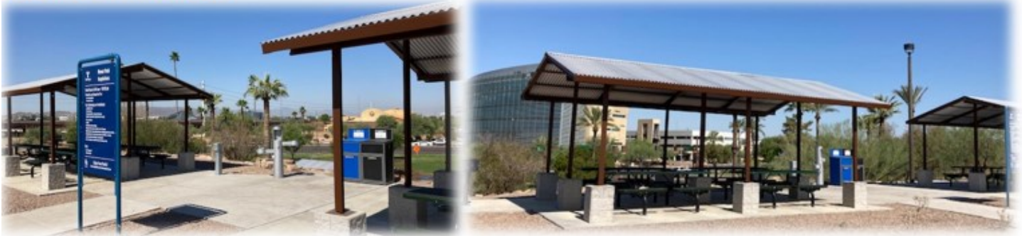
Above: Moeur Park Ramada Restoration & Renovation
