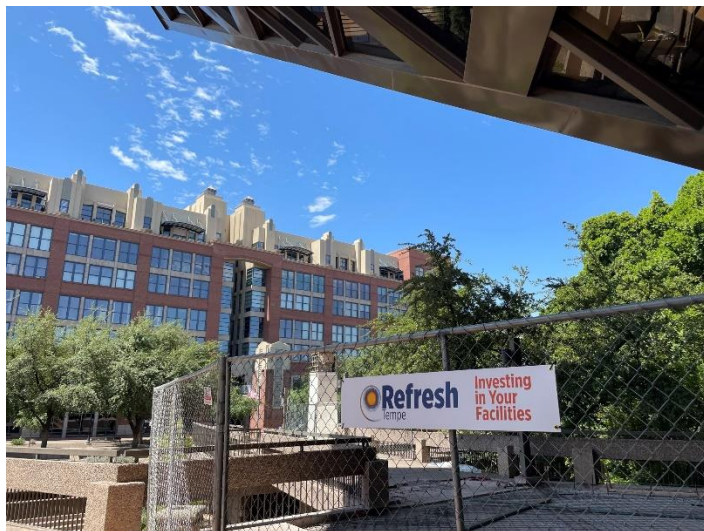
City Hall deck construction
