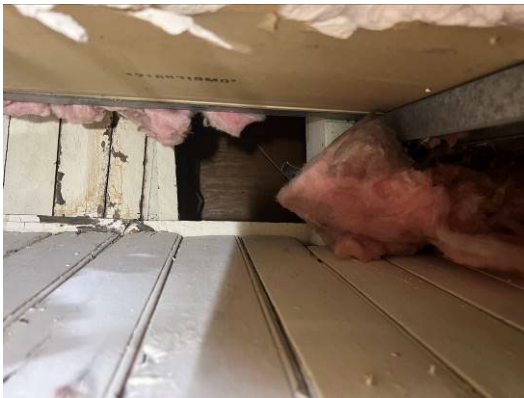
View upward in north wall cavity to ceiling
