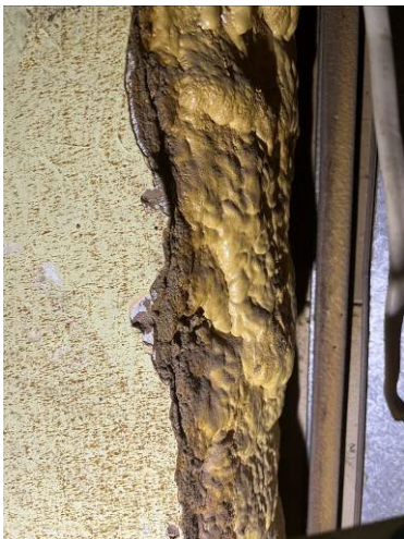
Adobe wall patched with polyurethane foam
