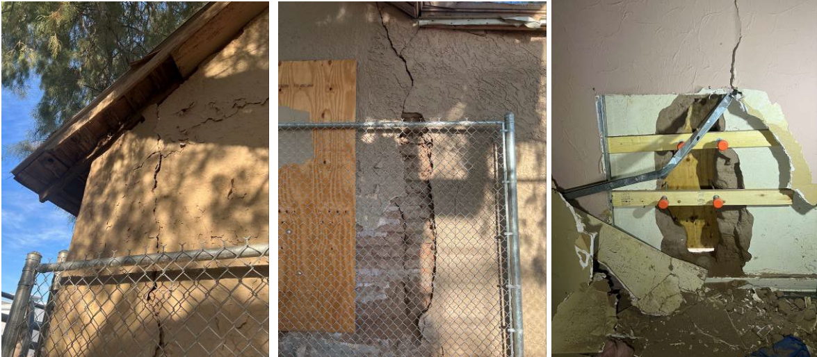
East wall condition
