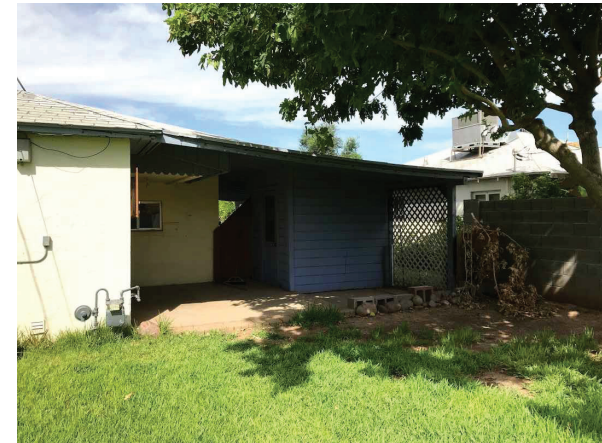
BACK PATIO - NE CORNER STRUCTURE
