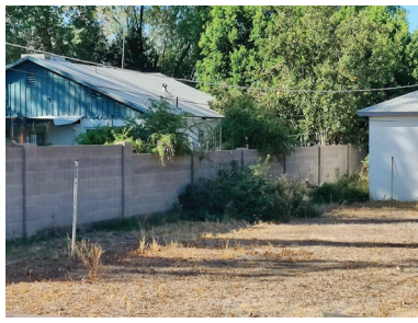
EXISTING NEIGHBOR SOUTH WALL
