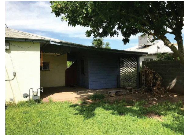
BACK PATIO - NE CORNER STRUCTURE
