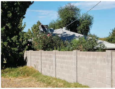
EXISTING NEIGHBOR NORTH WALL
