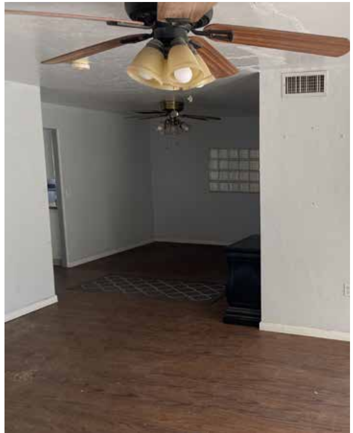
Existing light fixtures
