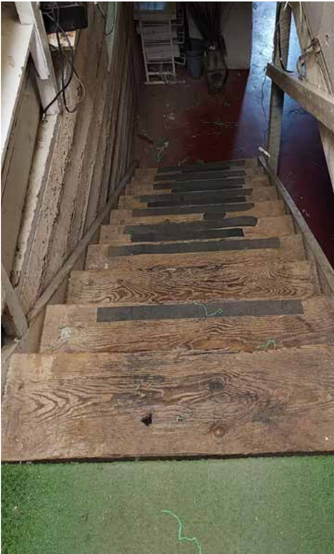
Basement stair down
