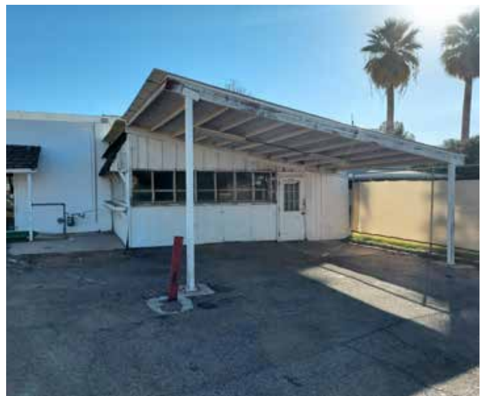
West building addition
