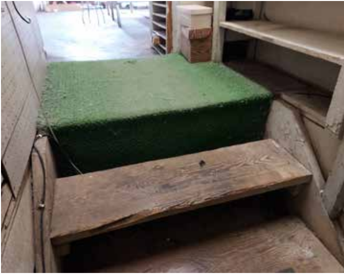
Basement stair landing
