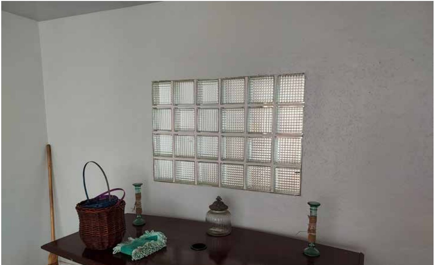
Glass block window - side 01
