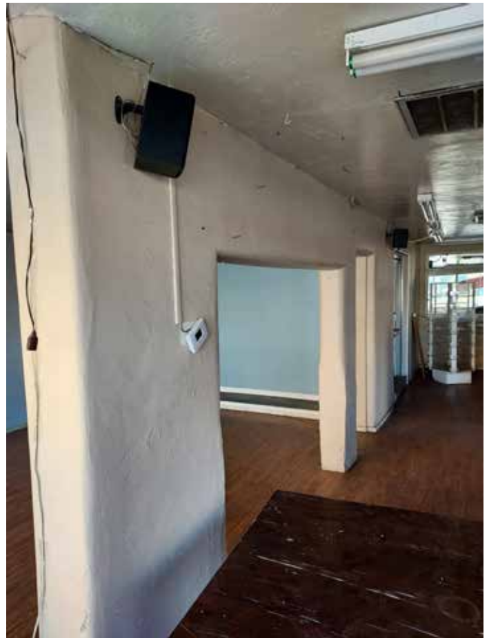
Interior bearing wall
