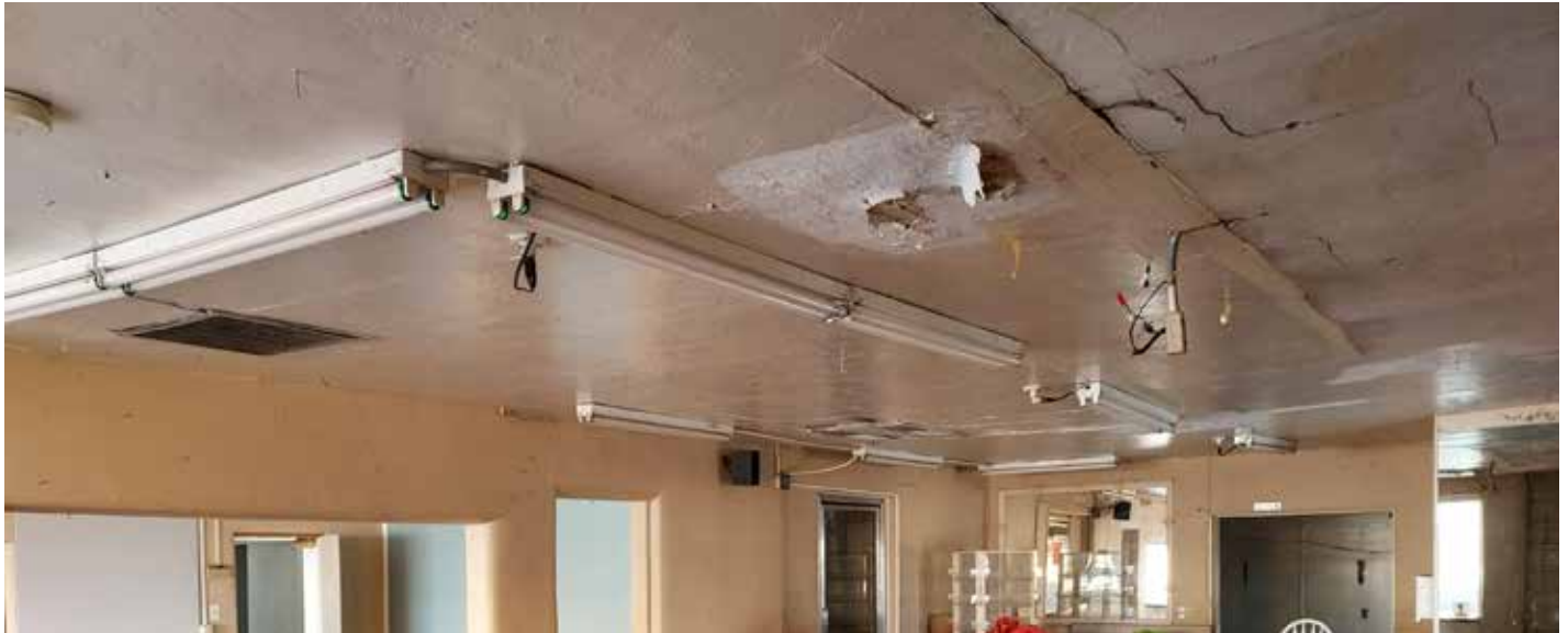
Sales room 01 ceiling
