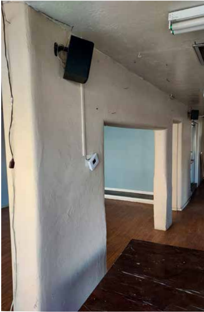
Interior remnant wall 01
