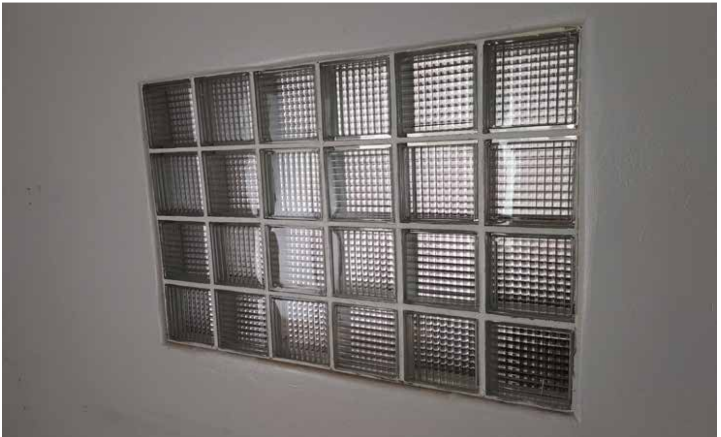
Glass block window - side 02
