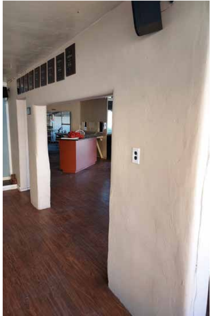
Interior remnant wall 02
