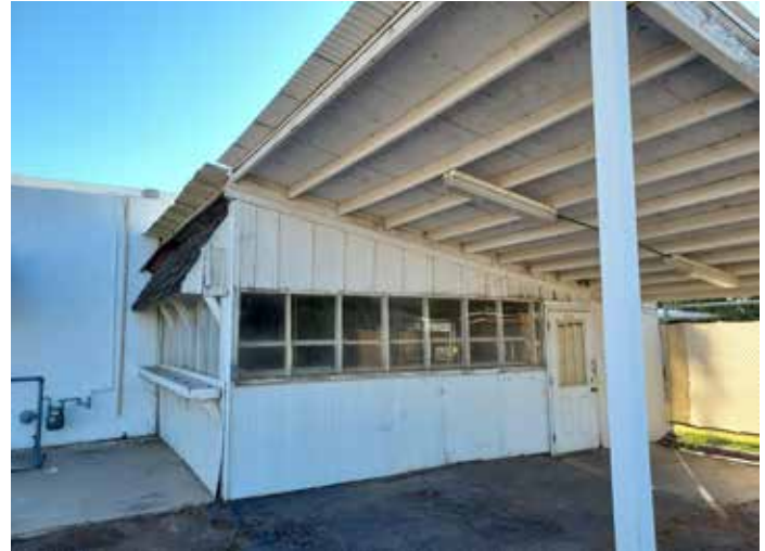
Late Addition on west side
