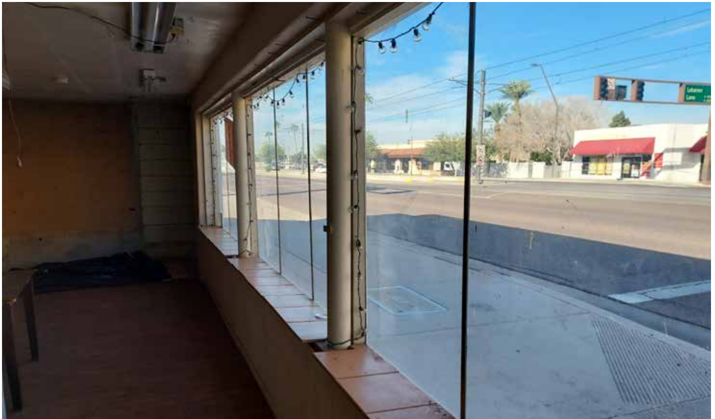
Pipe columns at W5
