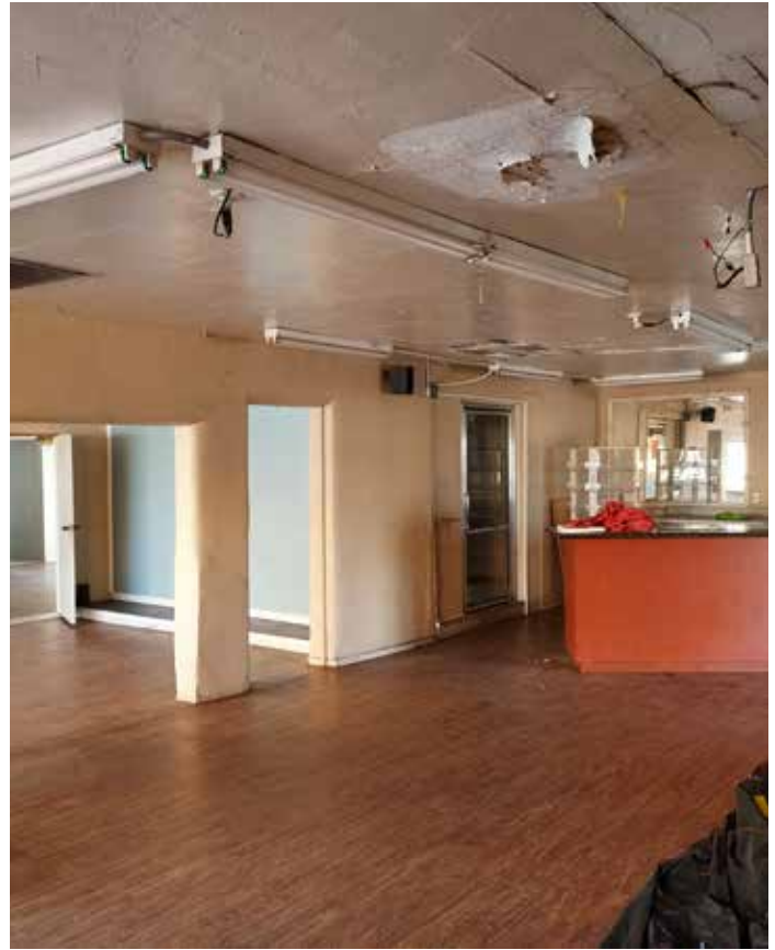
Existing light fixtures
