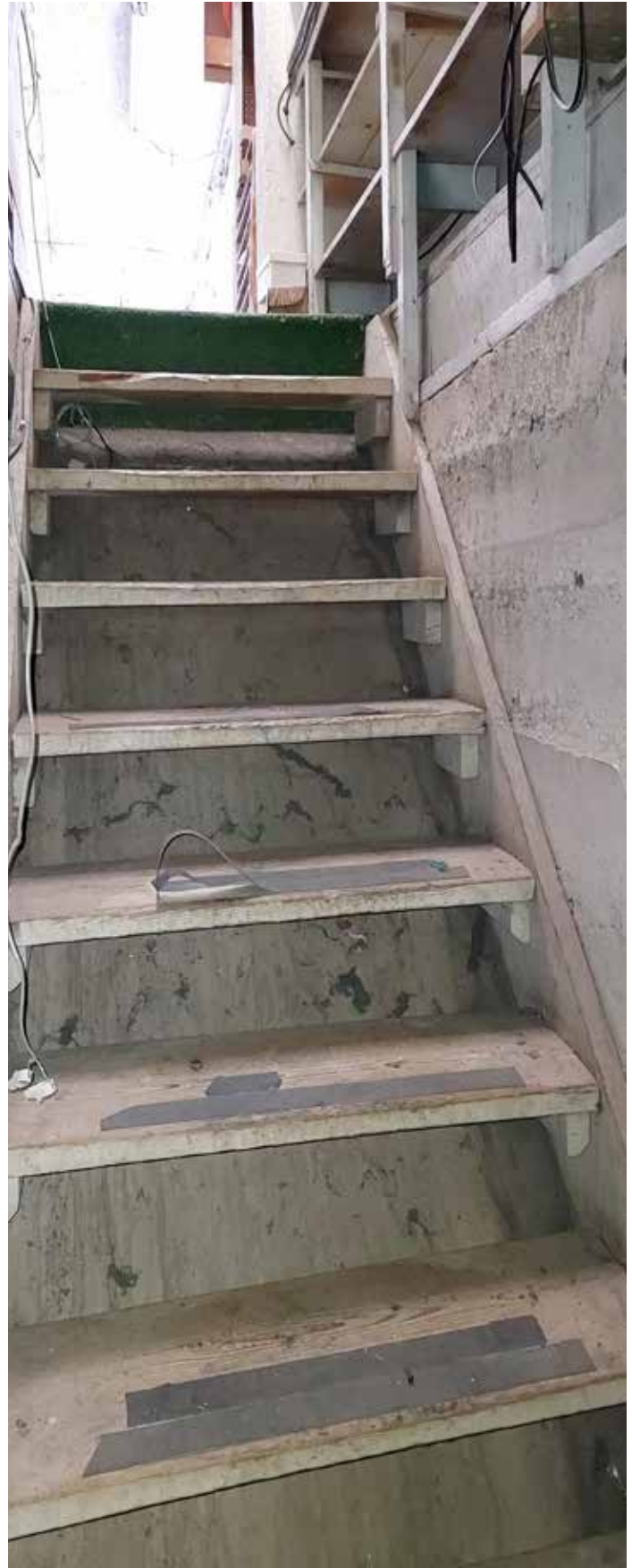
Basement stair up
