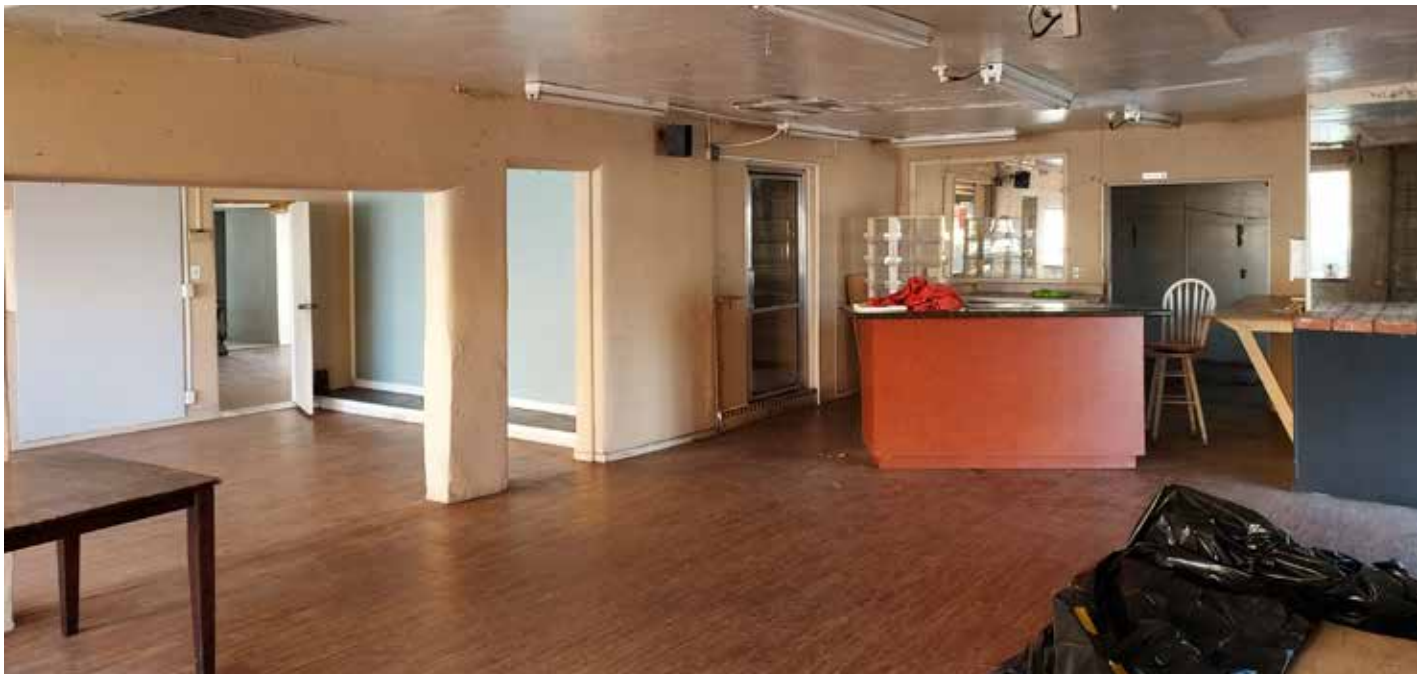
Interior remnant wall 02
