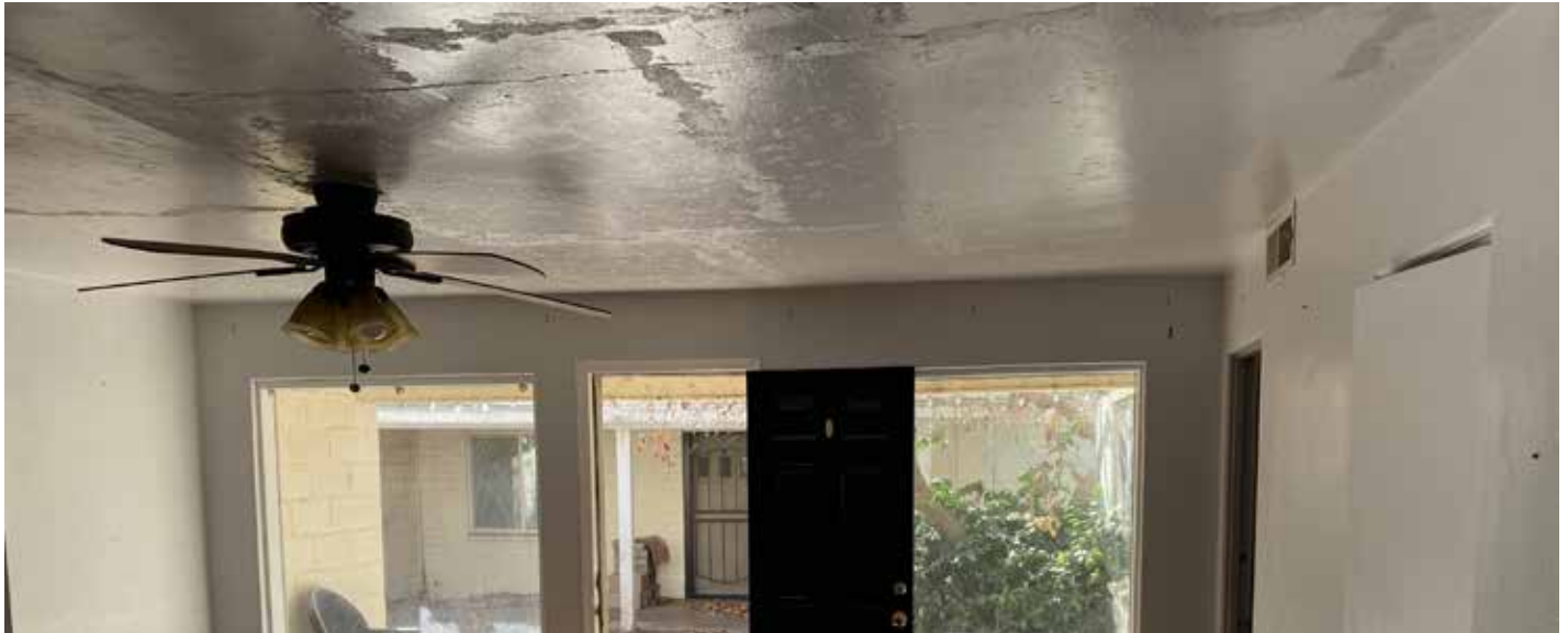
Living room 07 ceiling
