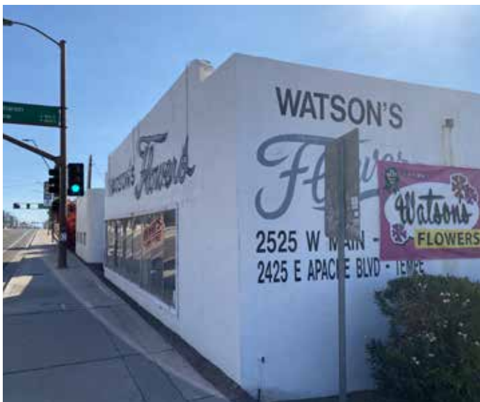
Northwest building corner
