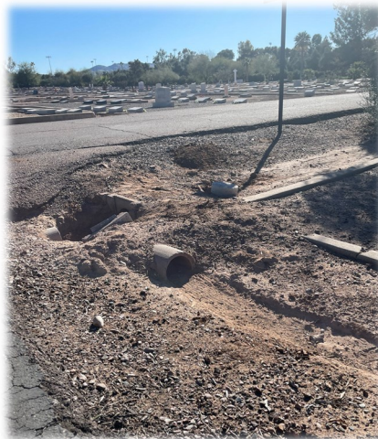
Irrigation ditch work
