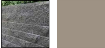
CMU-4 POP-OUT BLOCK ON EAST AND WEST SIDE OF BUILDING NEW (SUPERLITE) 8"x12"x16" SPLITFACE CMU SEMI GLOSS / COLOR: KEYSTONE GREY SHERWIN WILLIAMS TB24
