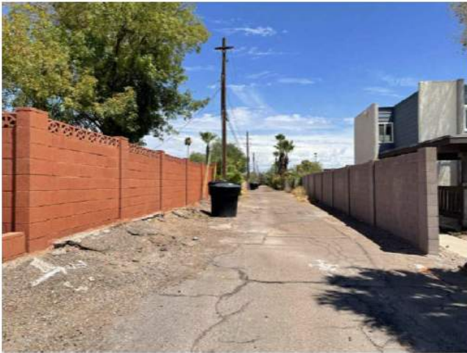
15 NW CORNER (LOOKING EAST)
