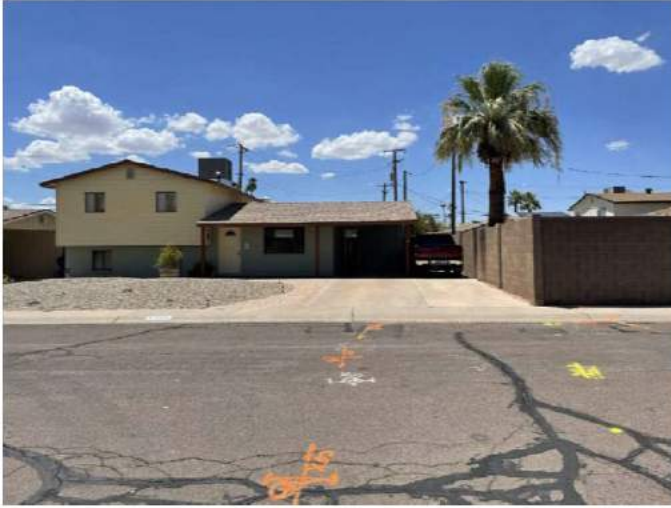
13 NW CORNER (LOOKING WEST)
