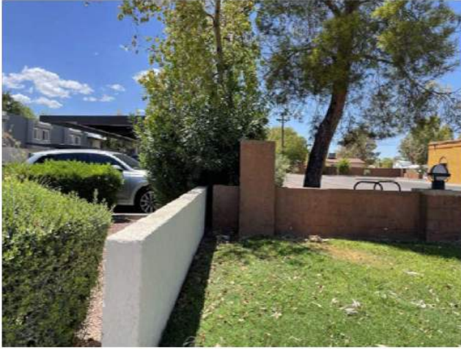
05 NE CORNER (LOOKING WEST)
