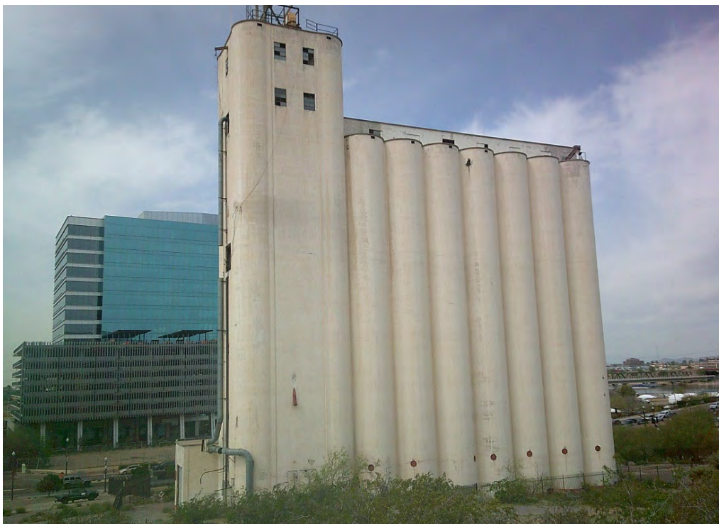
Photograph 10b. Overview of silos and grain elevators east elevation, view facing west (AZ_MaricopaCounty_HaydenFlourMill_010b)
