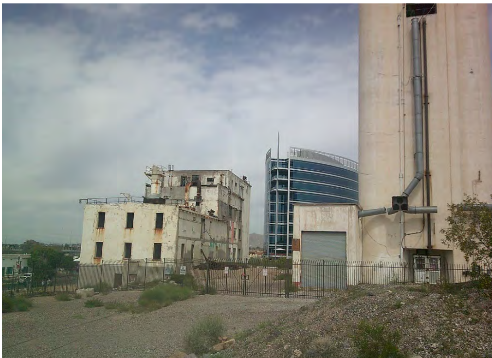
Photograph 10d. Detail of silos and grain elevators south elevation, view facing north-northwest (AZ_MaricopaCounty_HaydenFlourMill_010d)
