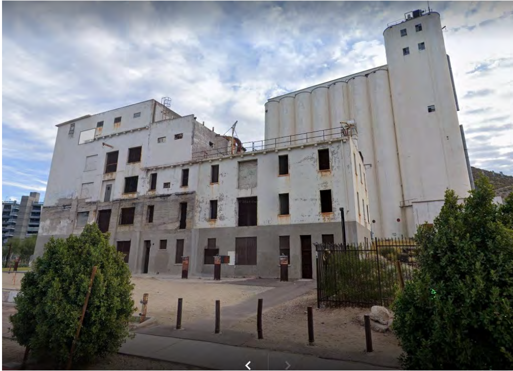
Photograph 2a. Overview of primary façade (west elevation) of the mill building taken from S. Mill Avenue, view facing west-northwest (AZ_MaricopaCounty_HaydenFlourMill_002a)
