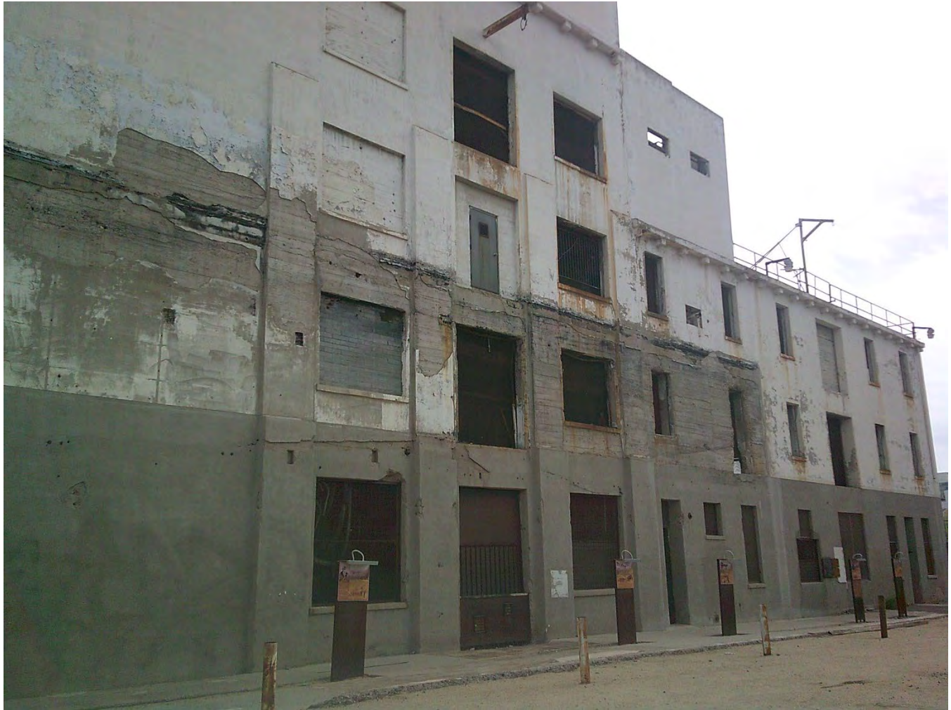
Photograph 3. Details of west elevation showing concrete pilasters and dentils along the parapet, view facing south-southeast (AZ_MaricopaCounty_HaydenFlourMill_003)
