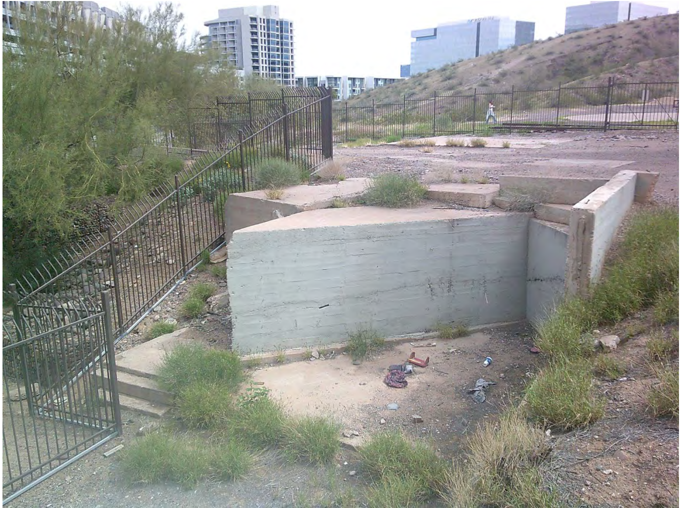
Photograph 12b. Resource No. 2, remnants of wooden addition and cribbed wood tower above conveyance tunnel, view facing northeast (AZ_MaricopaCounty_HaydenFlourMill_012b)
