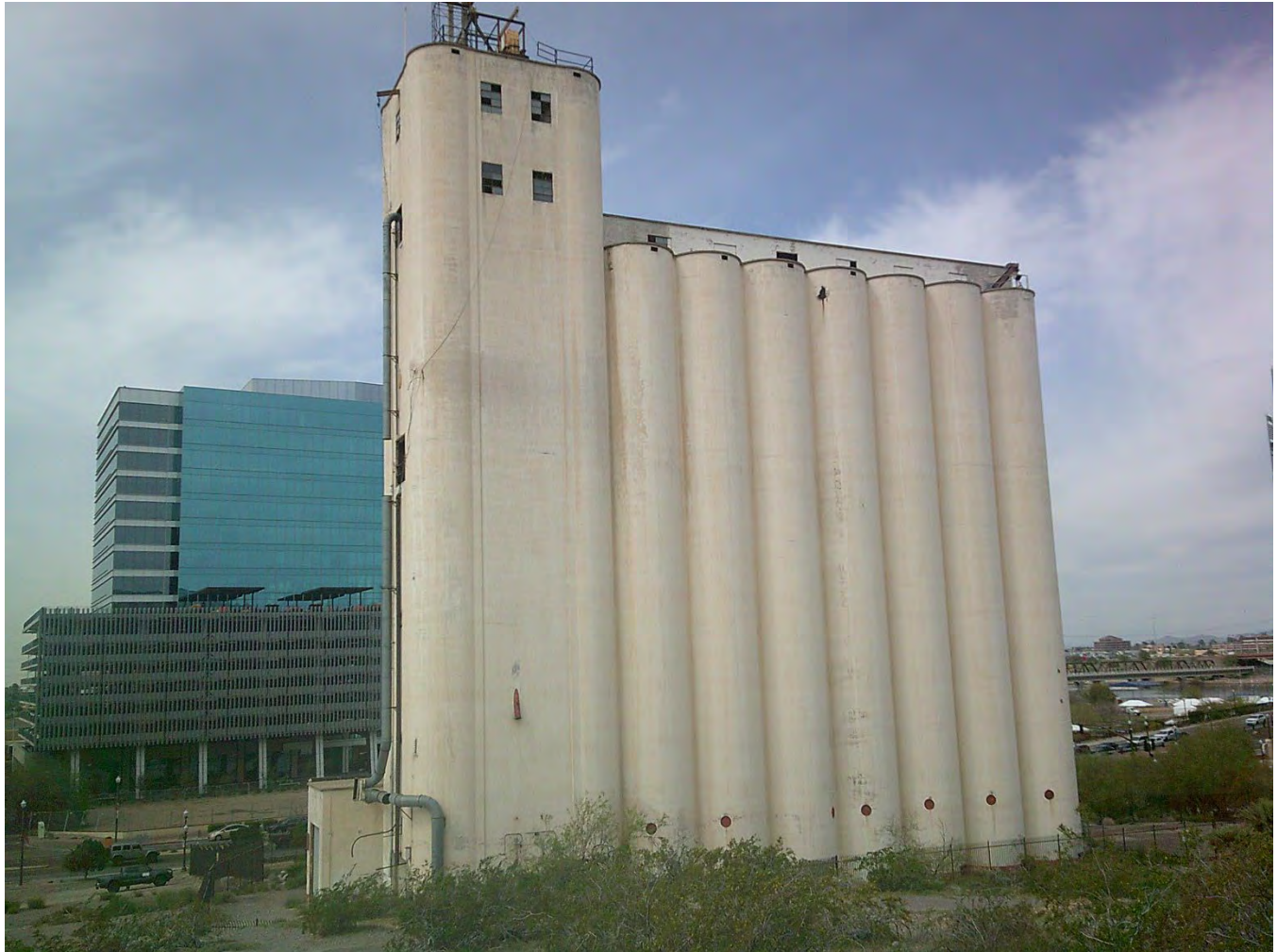
Photograph 10b. Overview of silos and grain elevators east elevation, view facing west (AZ_MaricopaCounty_HaydenFlourMill_010b)
