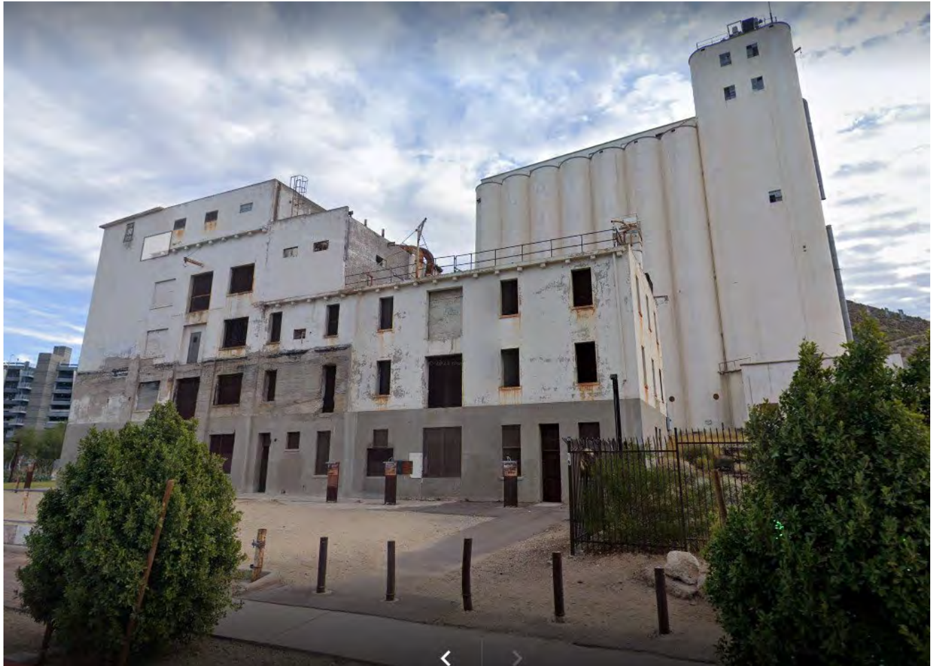
Photograph 2a. Overview of primary façade (west elevation) of the mill building taken from S. Mill Avenue, view facing west-northwest (AZ_MaricopaCounty_HaydenFlourMill_002a)
