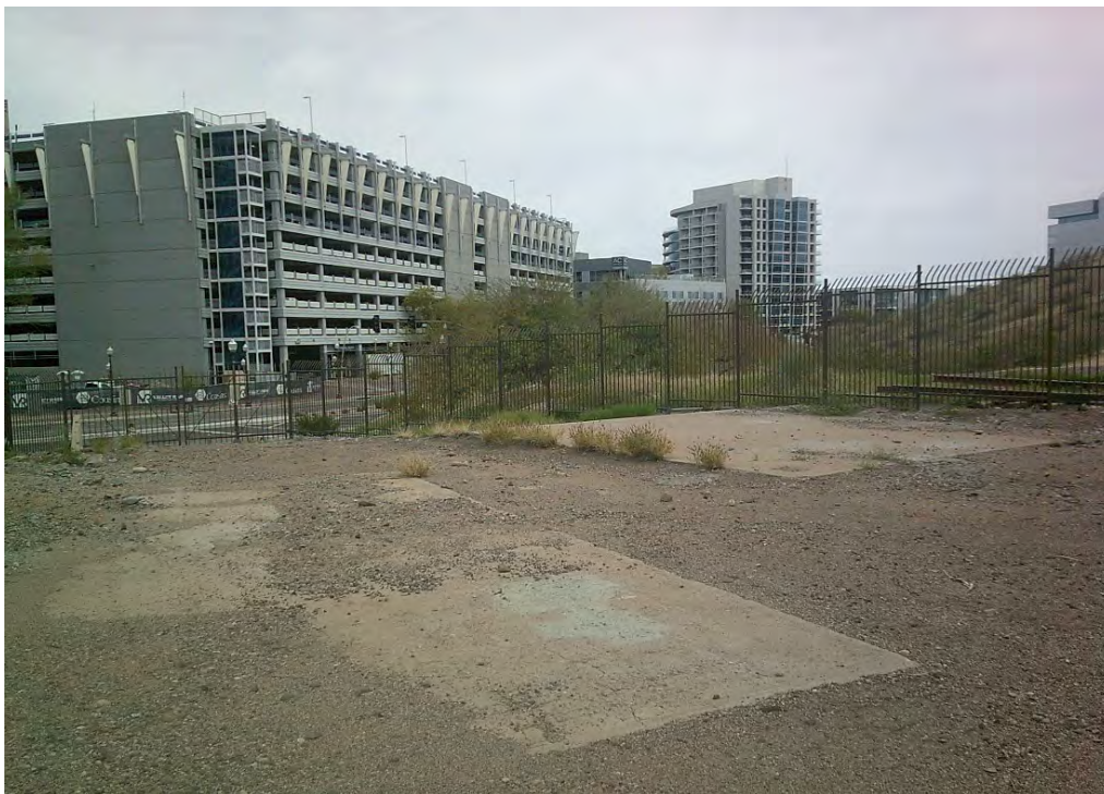
Photograph 13. Resource No. 3, shed foundations, facing north (AZ_MaricopaCounty_HaydenFlourMill_013)
