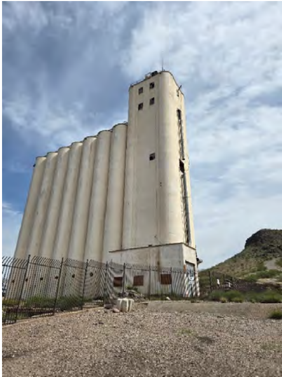
Photograph 10a. Overview of silos and grain elevators west elevation with Tempe Butte in background, view facing east-northeast (AZ_MaricopaCounty_HaydenFlourMill_010a)
