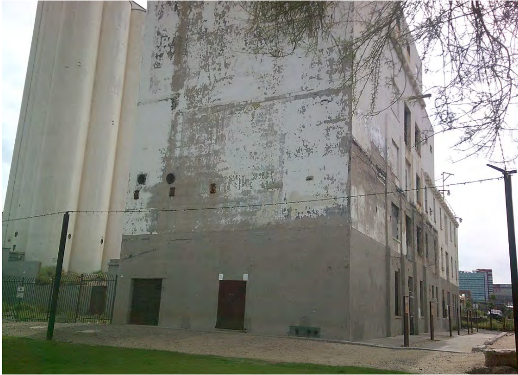
Photograph 2c. Overview of north elevation of mill building, view facing southeast (AZ_MaricopaCounty_HaydenFlourMill_002c)
