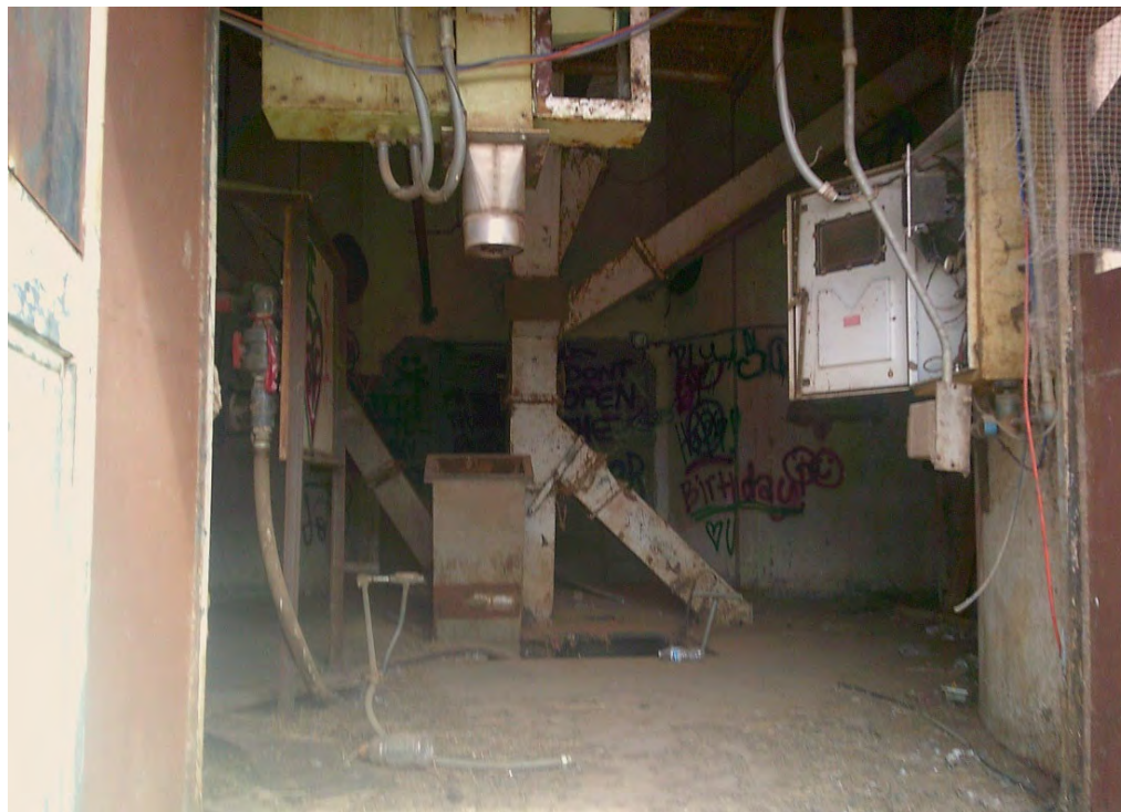
Photograph 14. Interior of ground floor of grain elevator, view facing north (AZ_MaricopaCounty_HaydenFlourMill_014)
