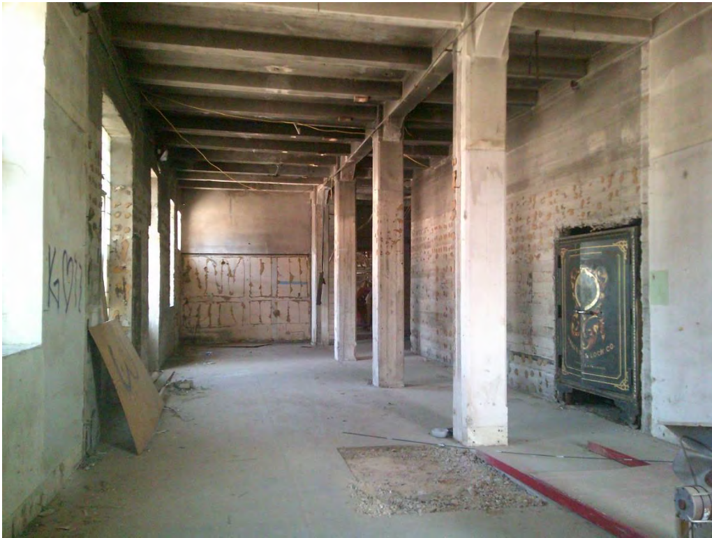
Hayden Flour Mill, 1918 building interior first floor, view facing north (WestLand Engineering & Environmental Services, March 14, 2024)
