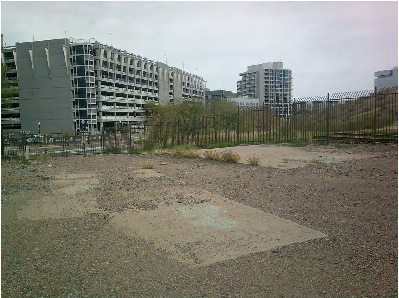
Photograph 13. Resource No. 3, shed foundations, facing north (AZ_MaricopaCounty_HaydenFlourMill_013)
