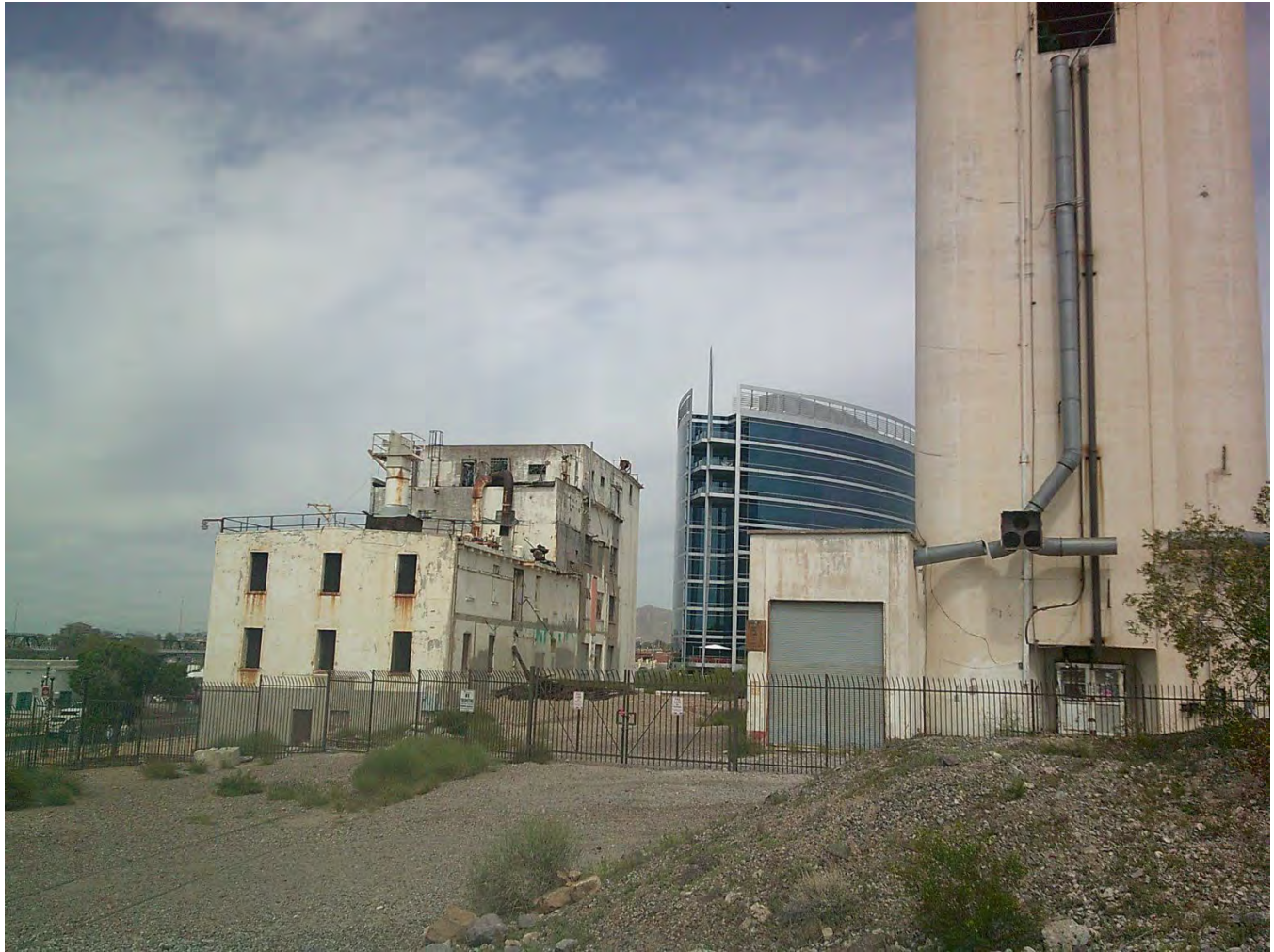
Photograph 10d. Detail of silos and grain elevators south elevation, view facing north-northwest (AZ_MaricopaCounty_HaydenFlourMill_010d)
