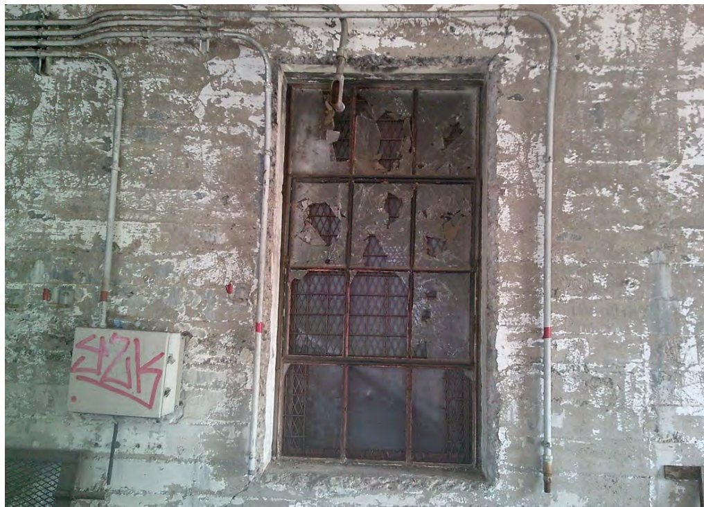
Photograph 4. Example of original window on east elevation, view facing east (AZ_PimaCounty_HaydenFlourMill_004)
