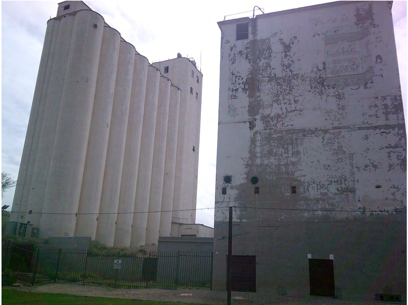
Photograph 10c. Overview of silos and grain elevators north elevation, view facing southeast (AZ_MaricopaCounty_HaydenFlourMill_010c)
