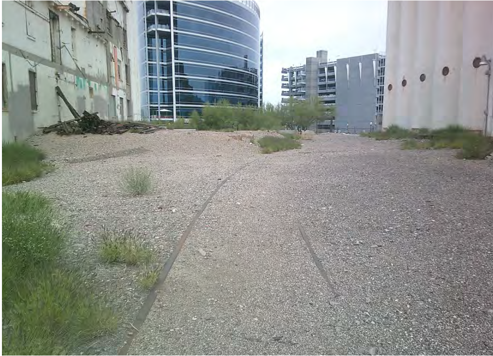
Photograph 11. Resource No. 1, former railroad spur, view facing north (AZ_MaricopaCounty_HaydenFlourMill_011)
