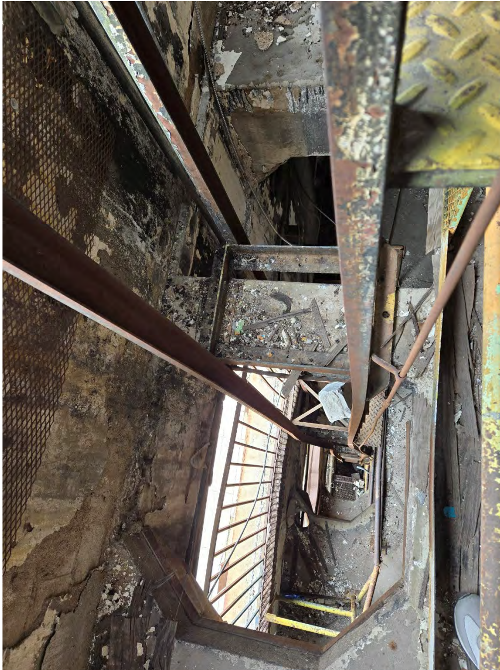
Photograph 8. View of manlift looking down from second floor (AZ_MaricopaCounty_HaydenFlourMill_009)
