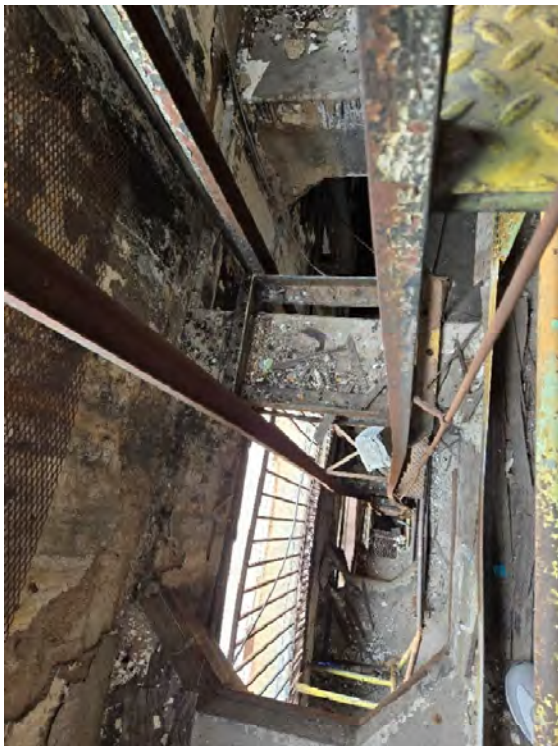
Photograph 8. View of manlift looking down from second floor (AZ_MaricopaCounty_HaydenFlourMill_008)
