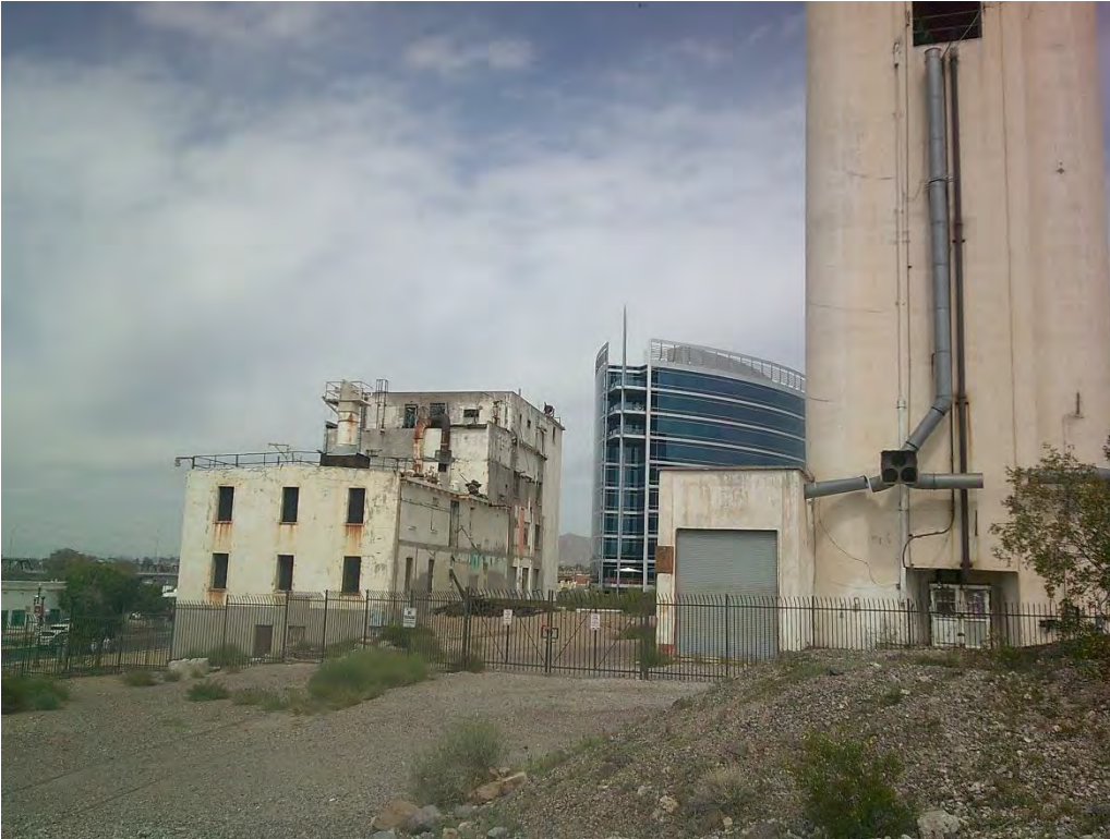
Hayden Flour Mill, overview of flour mill and grain silo, view facing north-northwest (WestLand Engineering & Environmental Services, March 14, 2024)
