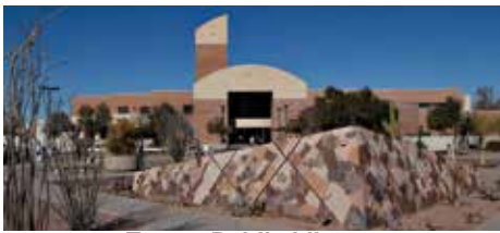
Tempe Public Library 3500 S. Rural Road 480-350-5500 • tempepubliclibrary.org
