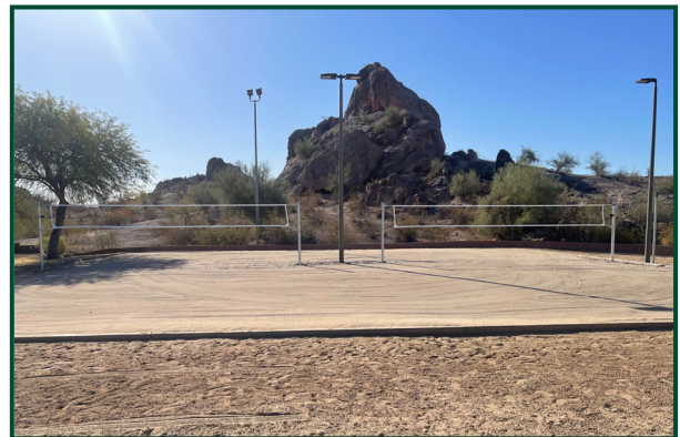
New sand installed at volleyball courts
