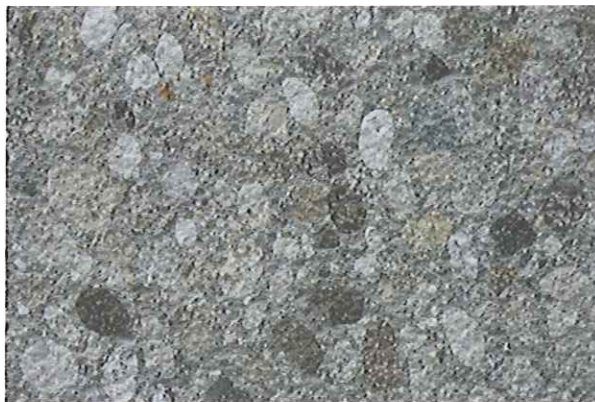
bushhammer concrete finish (selected site walls)
