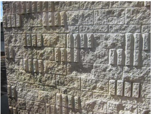
Split Faced, Textured Concrete Block Wall at Rural Road
