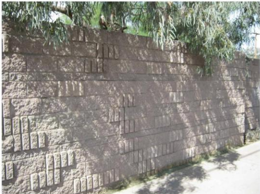
Split Faced, Textured Concrete Block Wall at Rural Road
