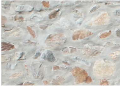
E LARGE AGGREGATE CONCRETE
