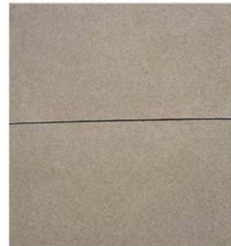
Acetate Finish Concrete
