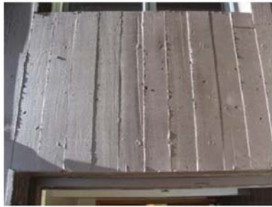
Board Formed Concrete
