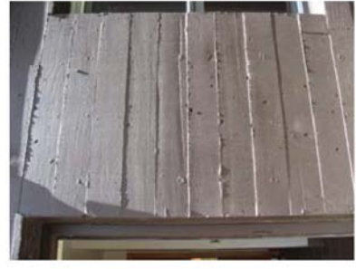
Board Formed Concrete
