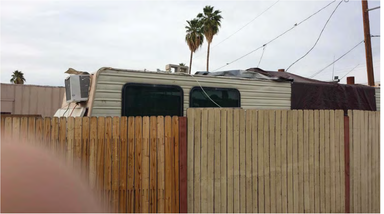
Picture #17: South End Facing North
