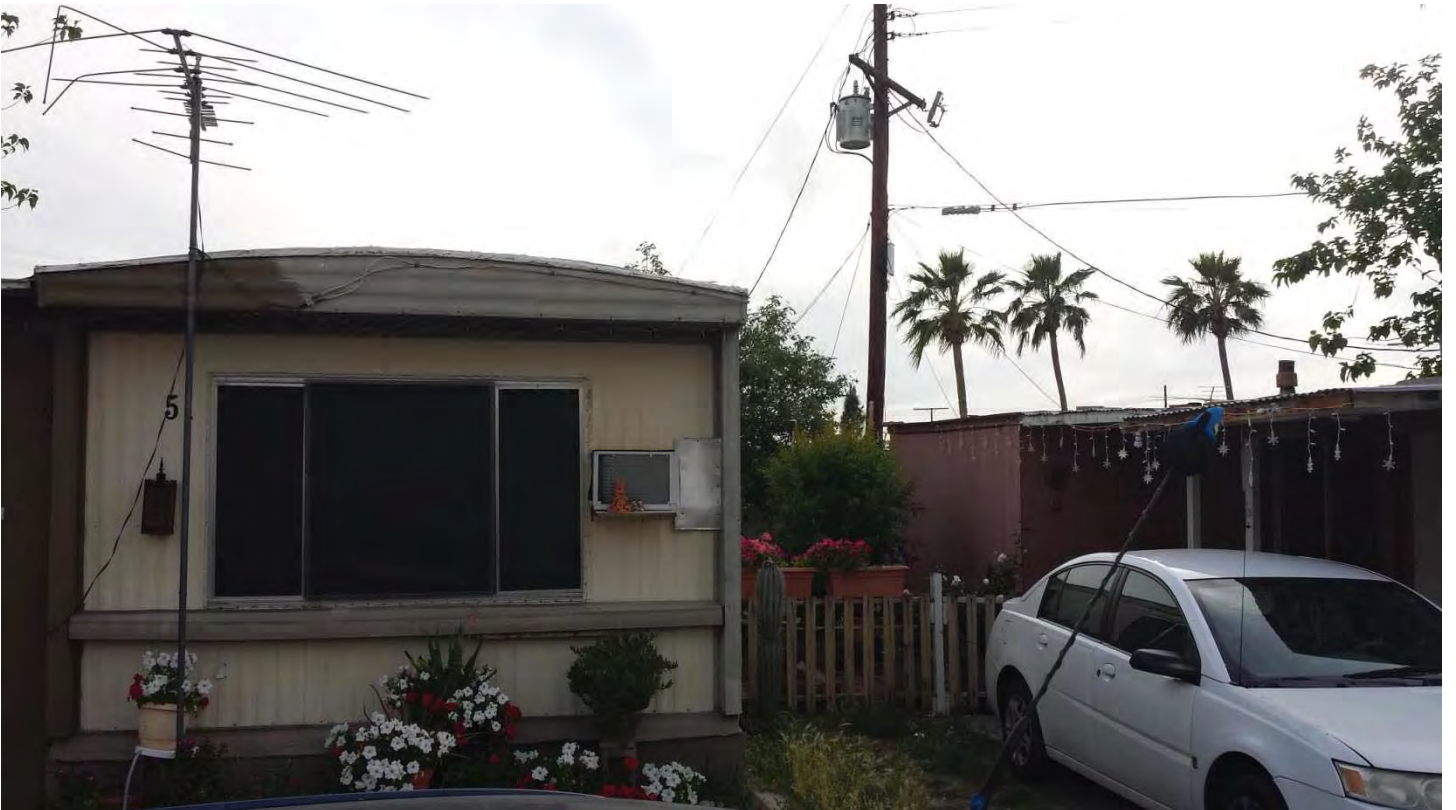
Picture #22: South End Facing Southwest
