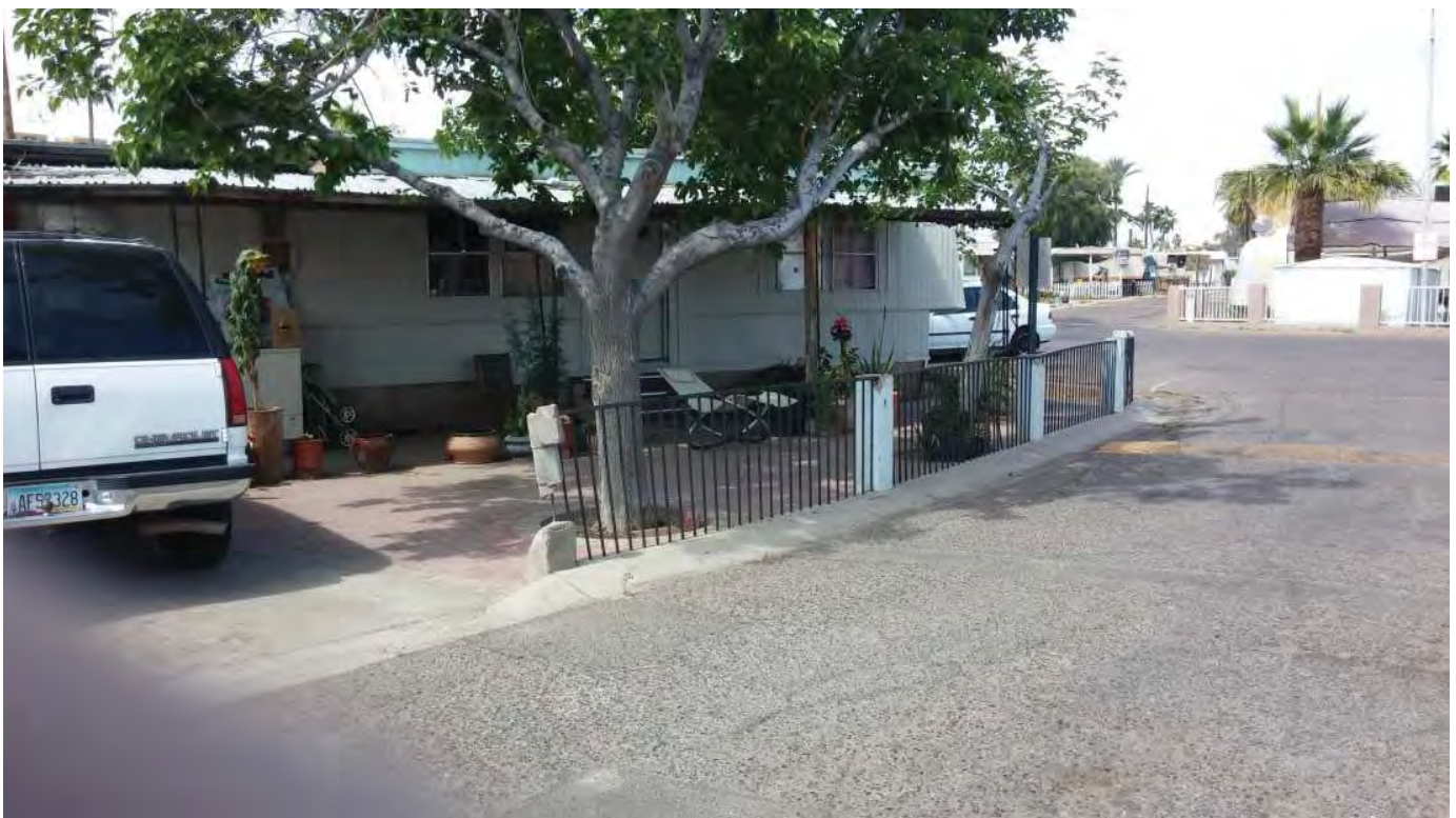
Picture #16: Center Facing Northwest
