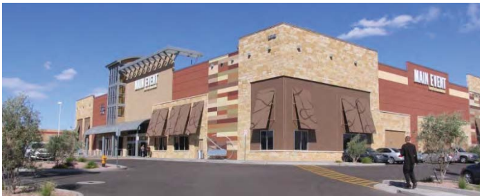
Main Event south west elevation looking north
