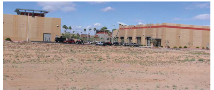
View looking north from site
