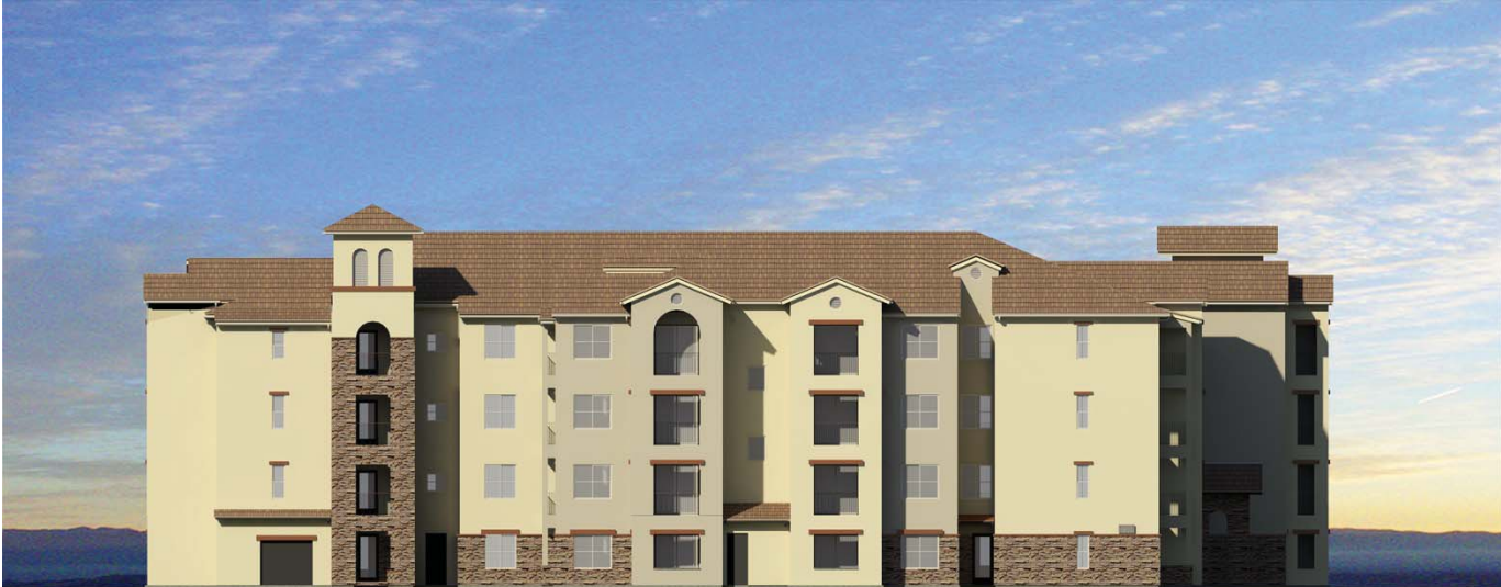
Apache Apartments north elevation
