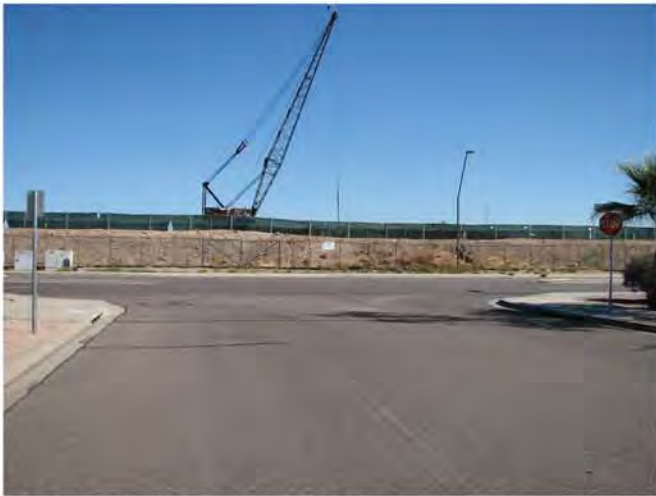
27 ROCKFORD DRIVE LOOKING NORTH SCALE: NTS
