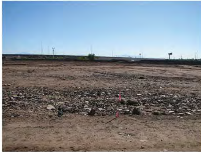
18 WEST SIDE LOOKING EAST SCALE: NTS
