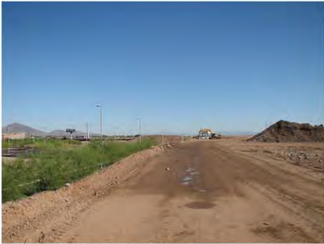
17 WEST SIDE LOOKING NORTH SCALE: NTS
