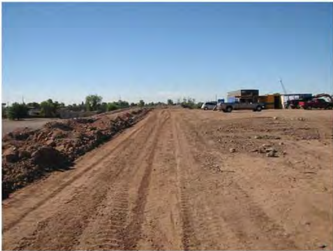
3 NEC LOOKING SOUTH SCALE: NTS
