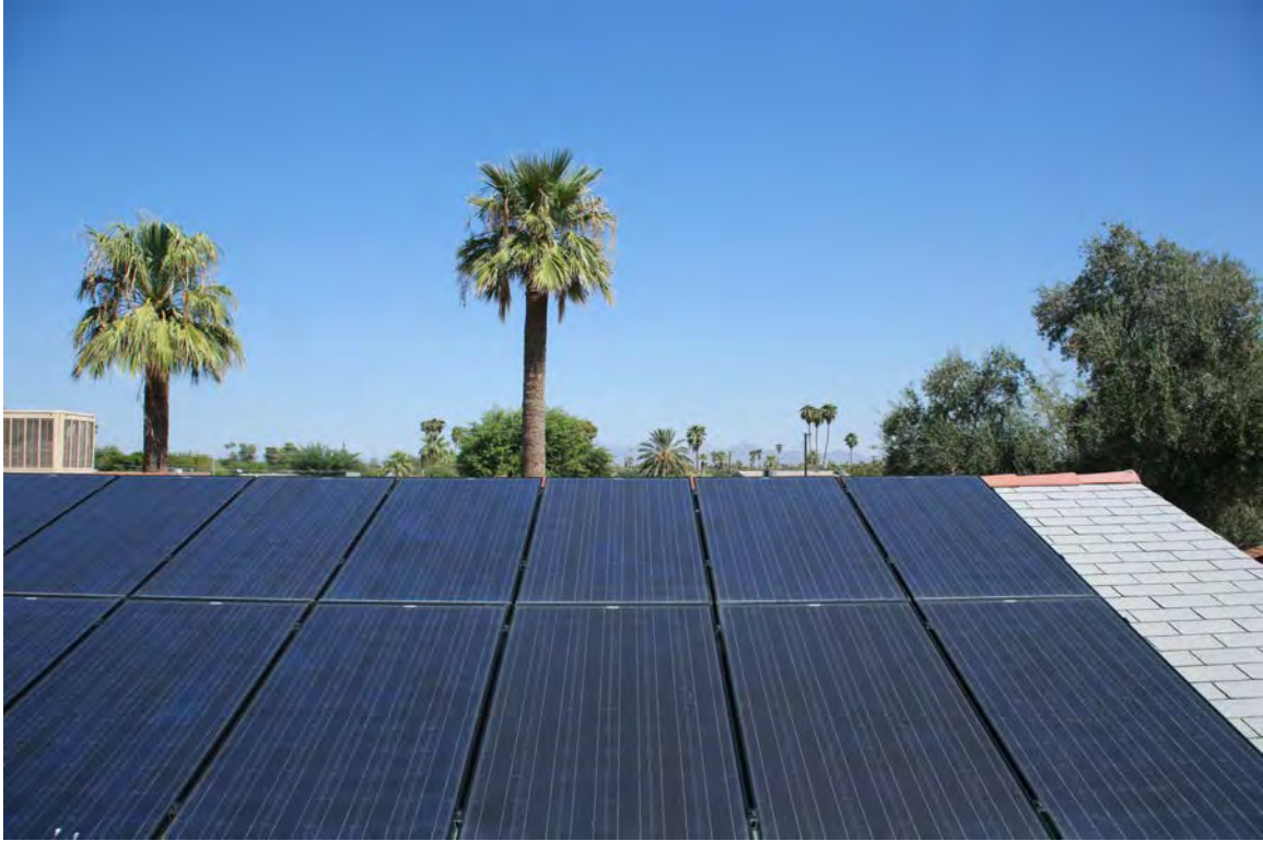
On the South Western edge of the deck facing North. Camera lens is at 5'8" above deck flooring. Street is NOT visible.
