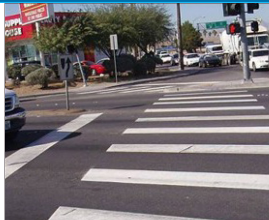
High-visibility crosswalks painted with reflective paint help motorists to see and yield sooner to people in the crosswalk.
