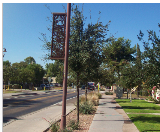
A sidewalk buffered with a landscape strip and a bike lane.
