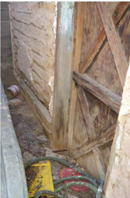
Exposed adobe wall segment (2014)
