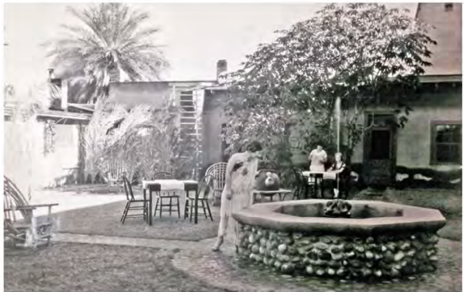
Interior courtyard, ca. 1925. The octagonal fountain was constructed as part of the Evans renovation project.
