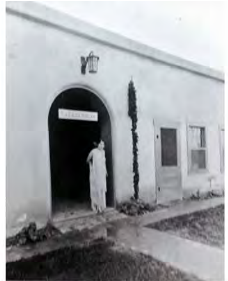
Archway, ca. 1925 on the north facade
