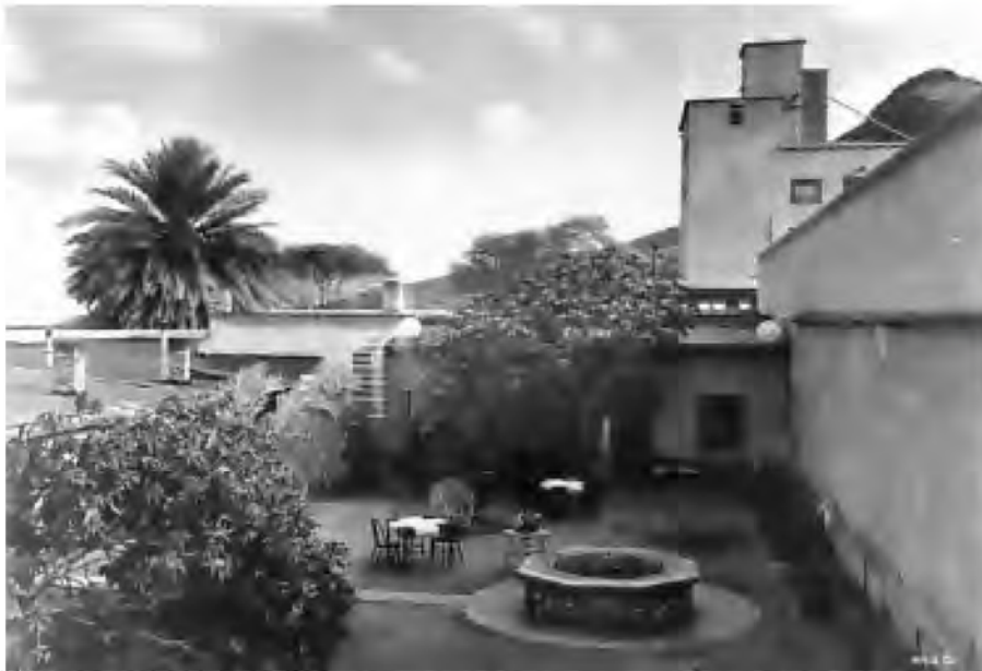
The Hayden House, ca. 1925; courtyard; view looking east. The flour mill rises in the background. The wall of the Hayden warehouse forms the courtyard wall to the south (right hand portion of the image).
