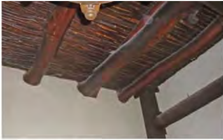
Detail of original ceiling (2014)
