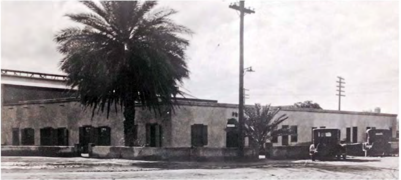
The Hayden House, ca. 1925, after the restoration by Robert T. Evans. Note the shutters on the windows. The Hayden warehouse rises behind.
