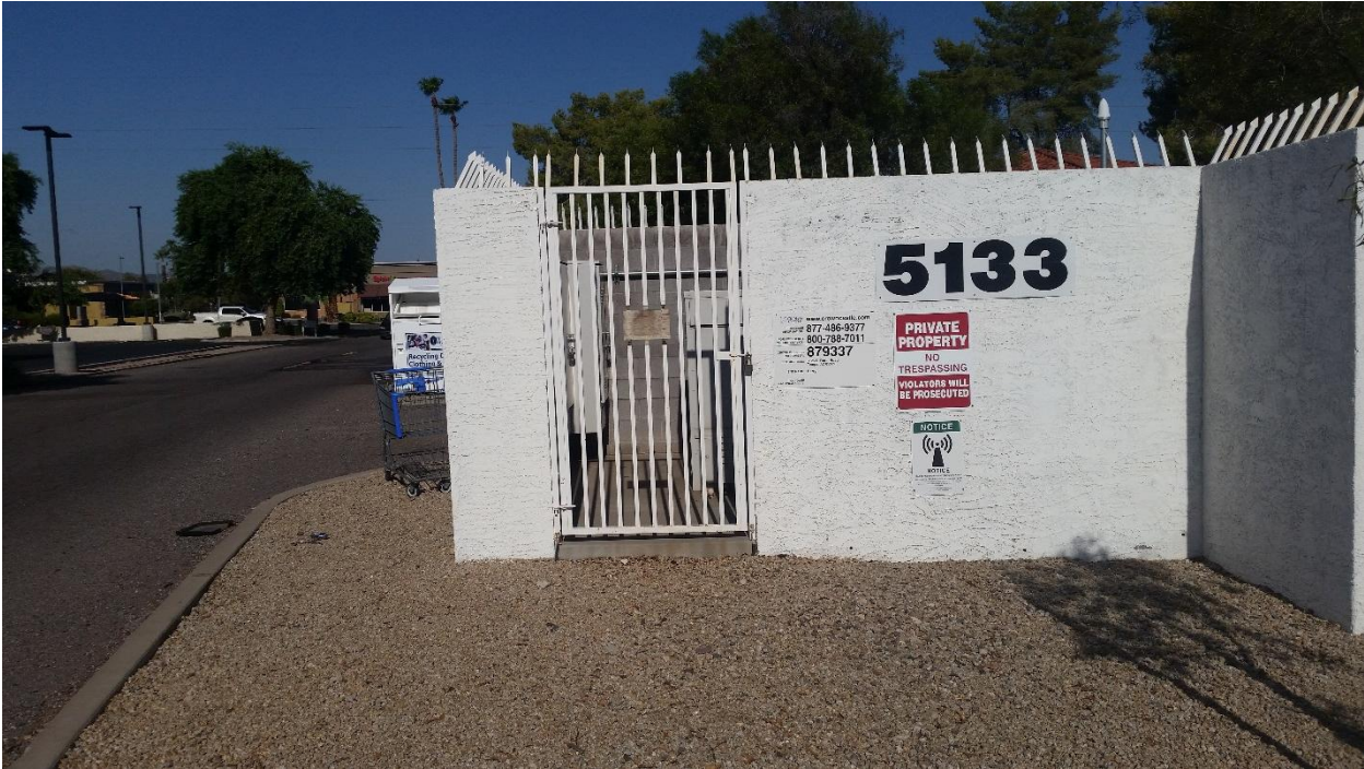
Photo 8: Southeast Corner (West)
