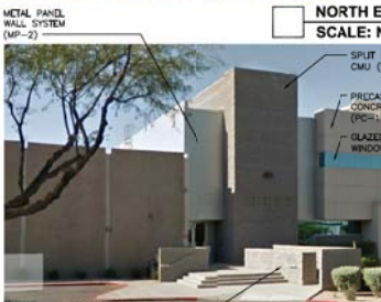
EXISTING FACILITIES PHOTOS SCALE: NONE
