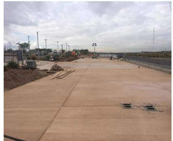
New sidewalk near the TCA
