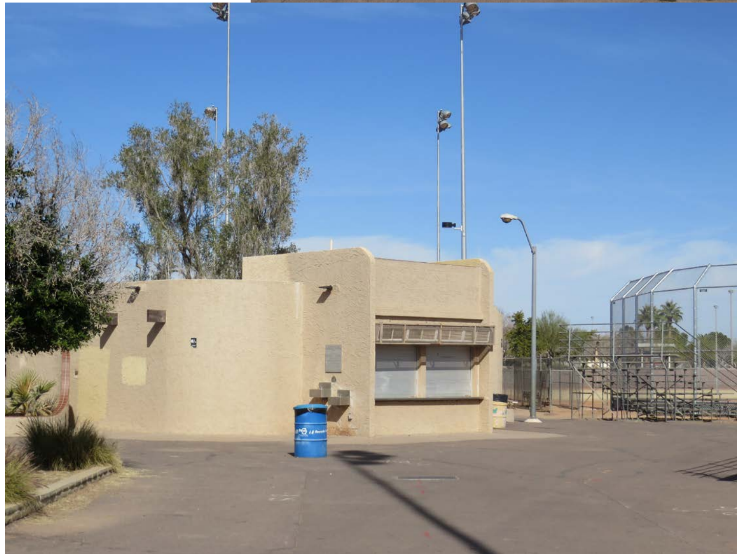
KIWANIS PARK Softball Complex Restroom Built c. 1977
