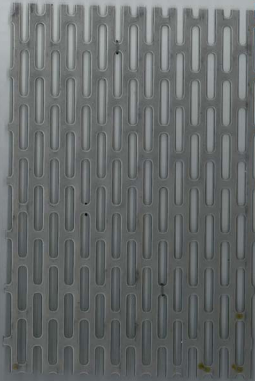
perforated metal panel: at garage
