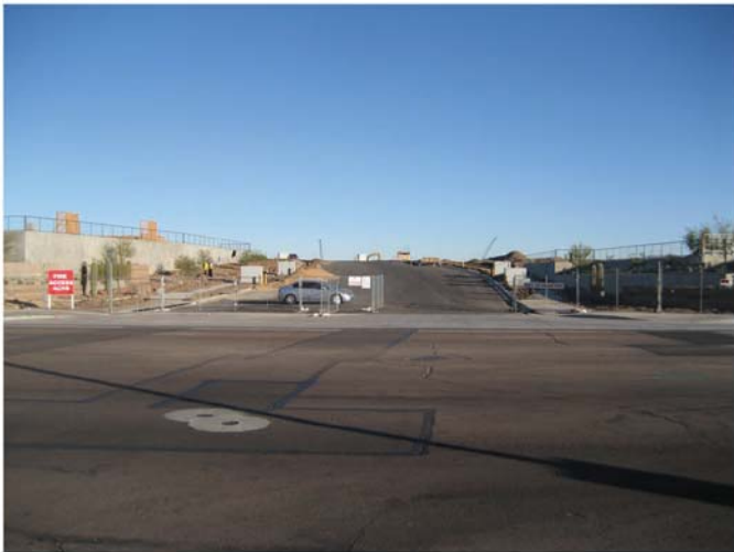
27 ROCKFORD DRIVE LOOKING NORTH SCALE: NTS
