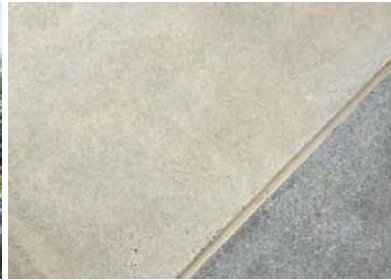
CIP CONCRETE PAVING
