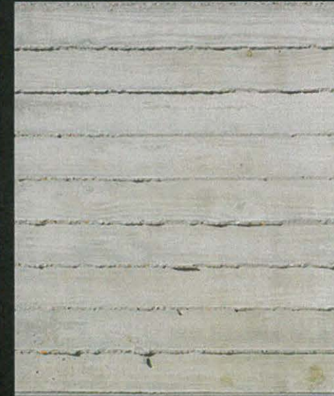
BOARD FORMED CONCRETE *
