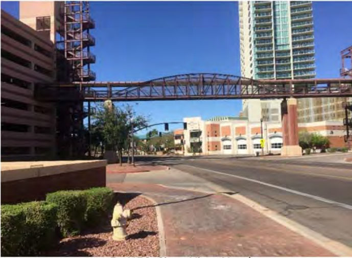
5. NEC Site - View North
