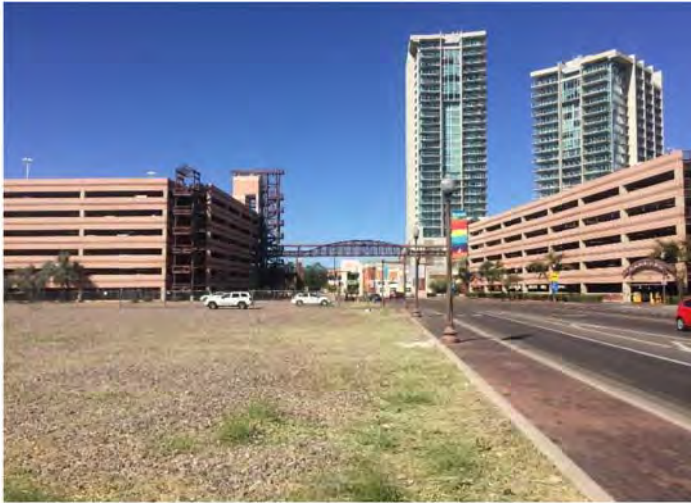
9. SEC Site - View North
