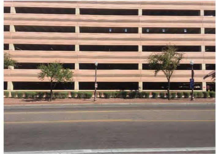
6. NEC Site - View East
