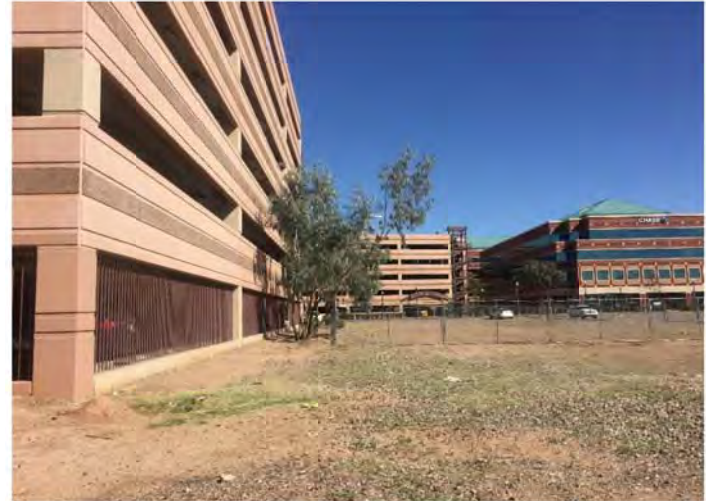
2. NWC Site - View East
