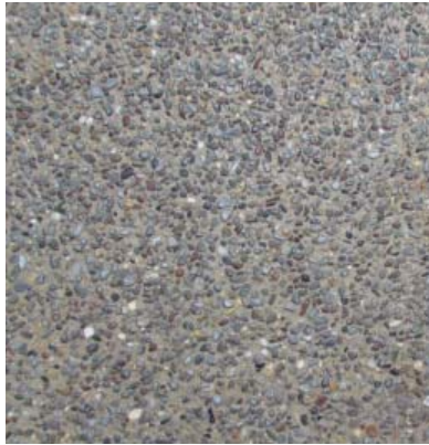
Decorative Concrete Paving: Exposed Aggregate
