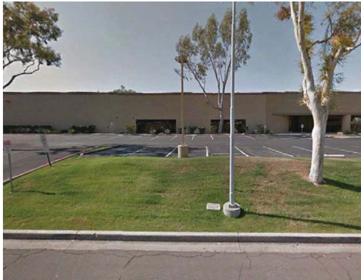
11. Location C (SWC) facing south
