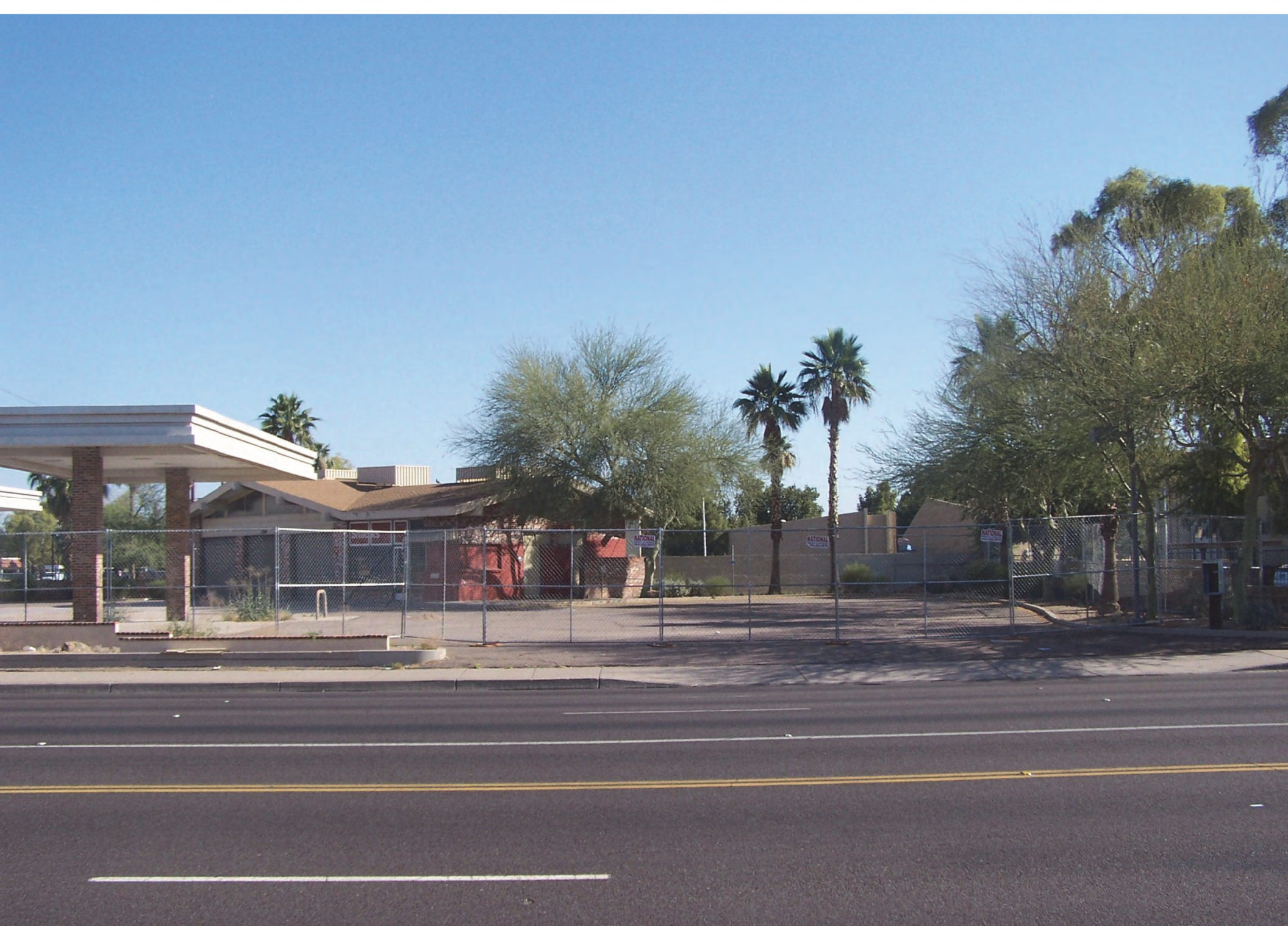
View from South (Denny's) looking towards Site
