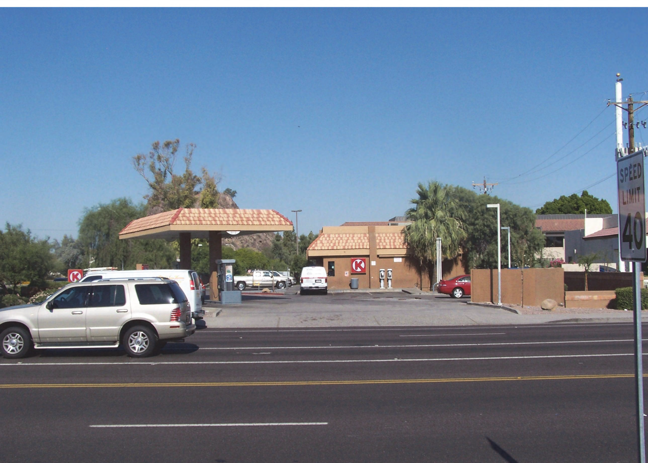
View from Site (south end) looking West at Convenience Mart
