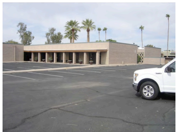
Photograph #28 South Mid-site looking NW
