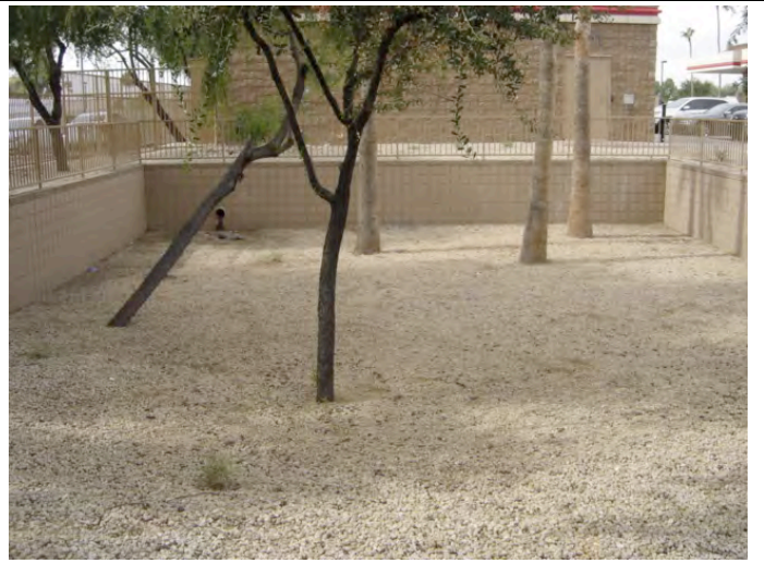
Photograph - East Retention
