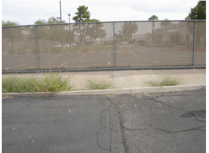
Photograph #32 South of South Mid-site looking East
