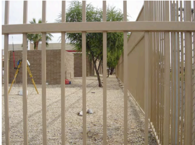
Photograph #31 South Mid-site looking East
