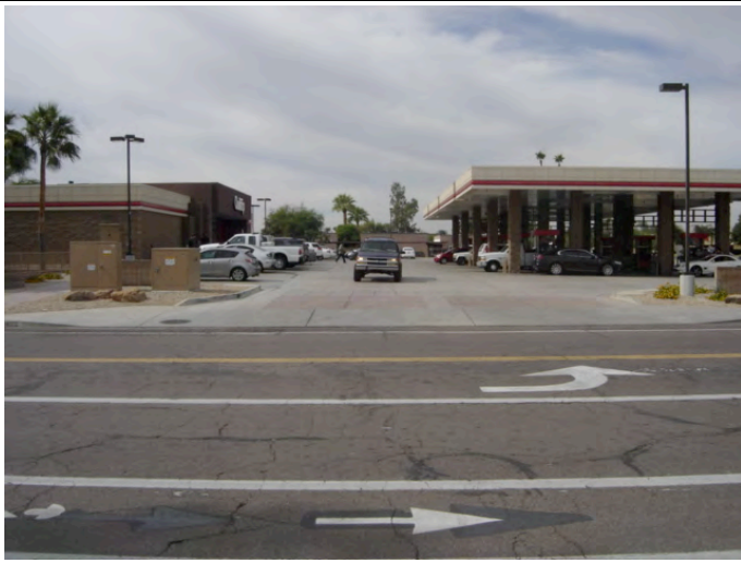
Photograph #41 Mid-site 52 nd Street looking West
