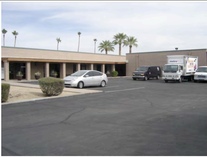
Photograph #23 SWC Hohokam Drive looking NE
