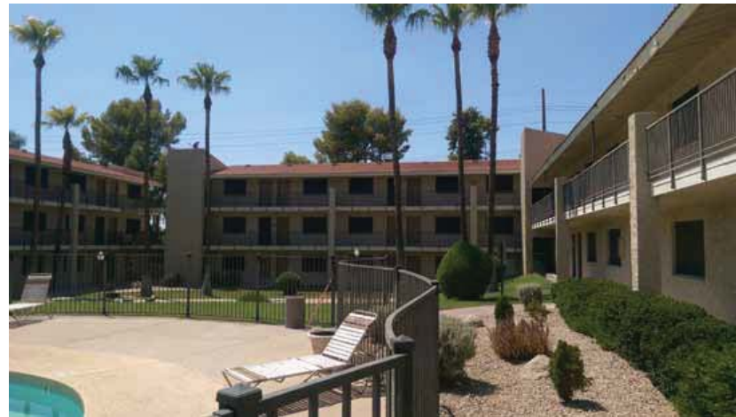
Interior Courtyard - looking west
