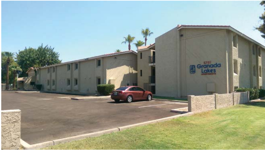
Existing Northwest building elevation along Rural Road and Southshore
