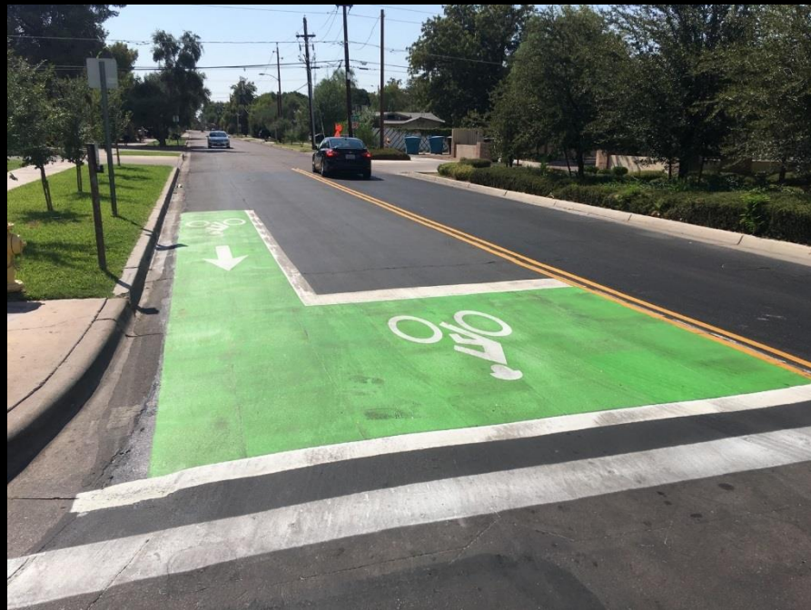
Bicycle Boxes at Intersections
