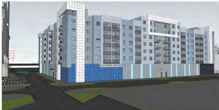
NORTHEAST CORNER VIEW
