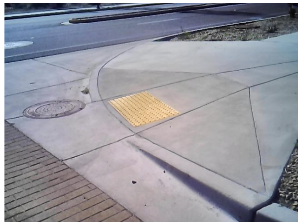
Figure 2: Compliant Perpendicular Ramp
