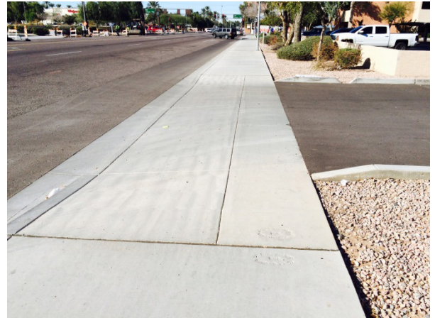
Figure 1: Accessible path behind driveway
