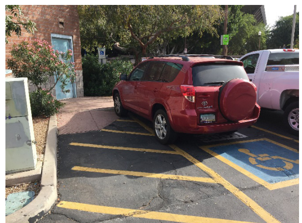
Figure 9: City Hall West - Curb Ramp within access aisle
