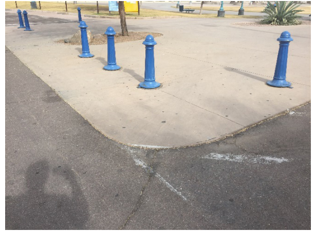
Figure 10: Change in level at access point
