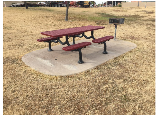
Figure 14: Corbell Park - No accessible route to amenities
