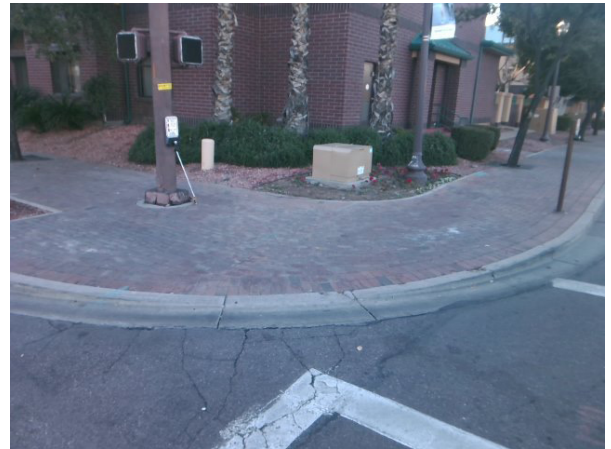
Figure 3: Install Detectable Warning System
