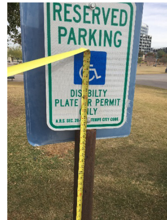
Figure 11: Parking signs are too low
