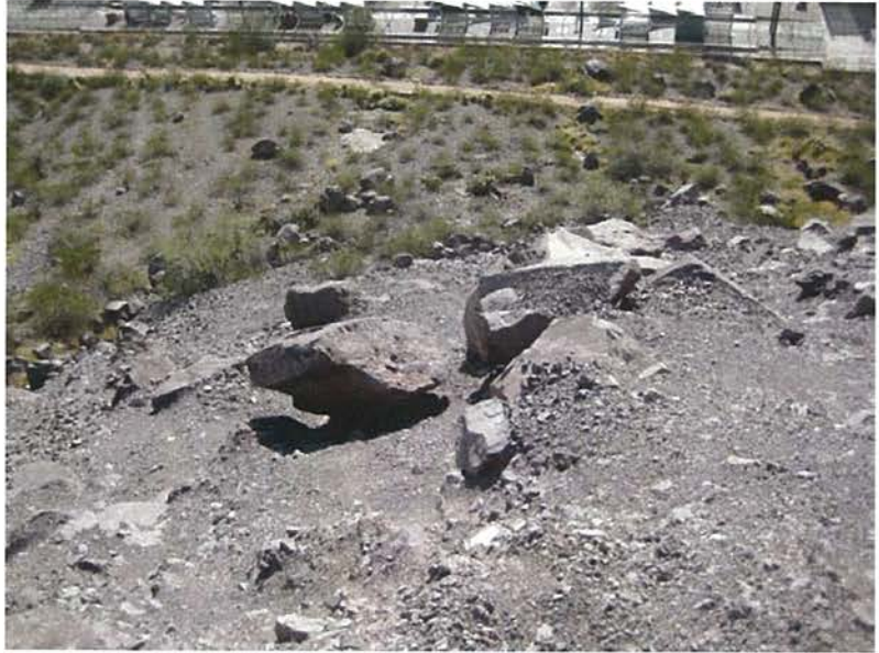
Photo 8: Loose boulders within the man-made tank excavation spoils.
