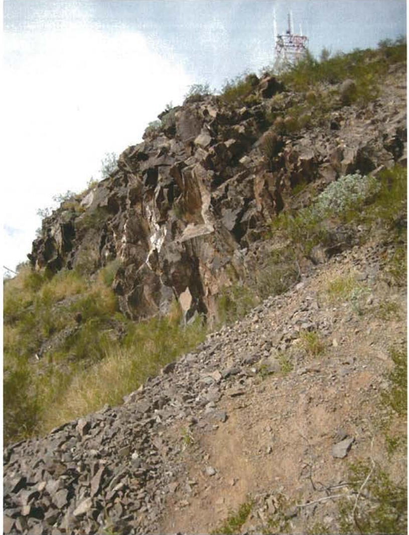
Photo 7: Loose boulders within the man-made tank excavation spoils.
