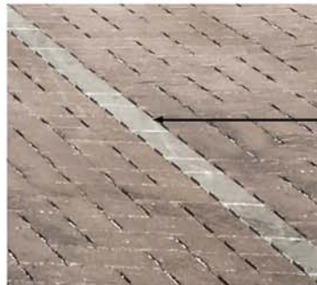
ACKERSTONE- HOLLAND STONE DAVIS COLOR: DARK GREY [PARKING STRIP] PRECAST PAVER, TYPE 2
