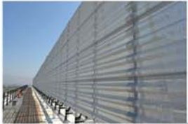
PERFORATED SCREEN WALL (EXAMPLE)
