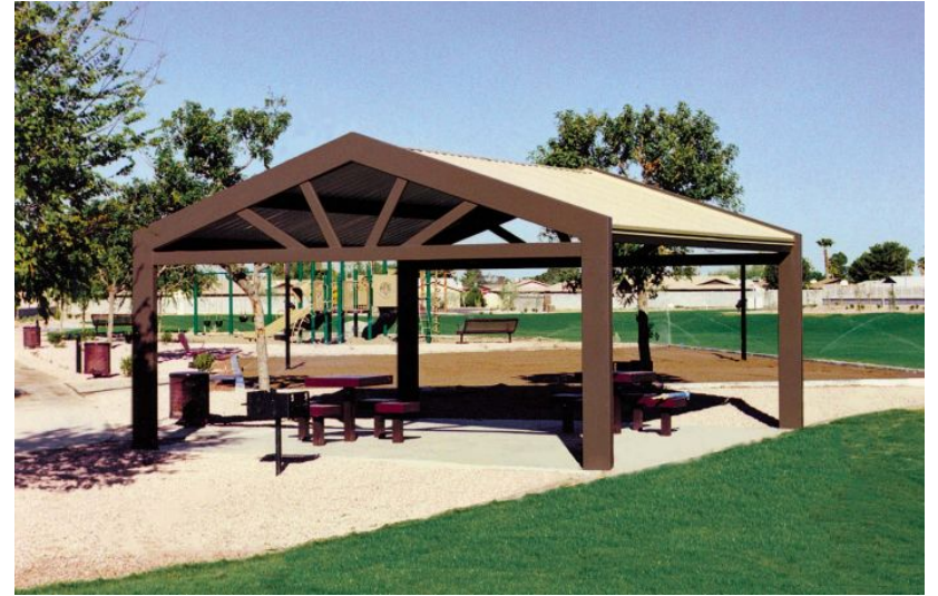
Metal Shade Structure
