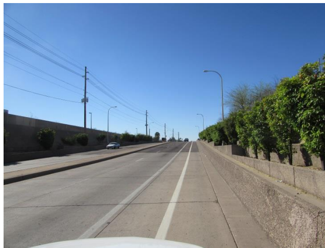
Example of trees affected in Alternative 3 along the west side of McClintock between Apache and Broadway.
