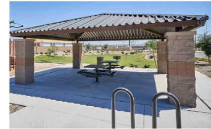
PICNIC RAMADA METAL ROOF STRUCTURE
