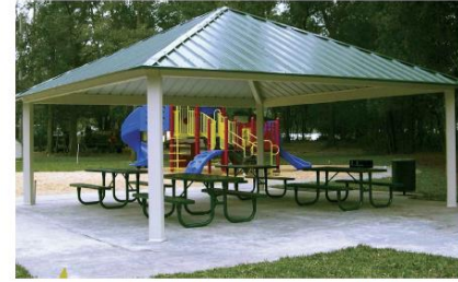
PICNIC RAMADA METAL ROOF STRUCTURE
