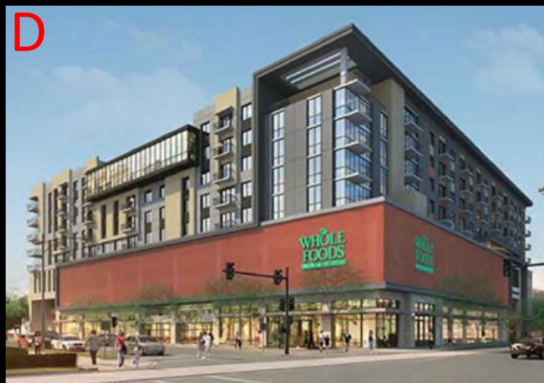
D The Foundry (Under Construction) Mixed Use – 9 Stories
