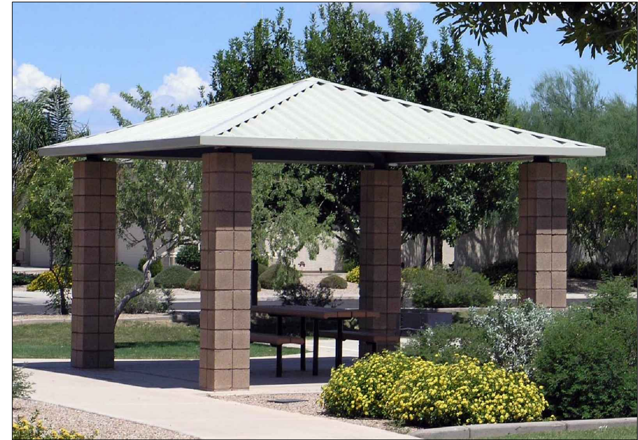
SCoured CMU BLOCK FINISH
